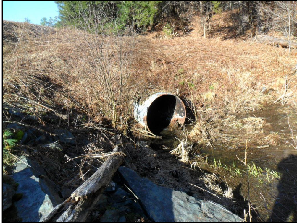
V-FH-S-10 Inlet of 42-in culvert located upstream from 48-in culvert proposed to be crossed
