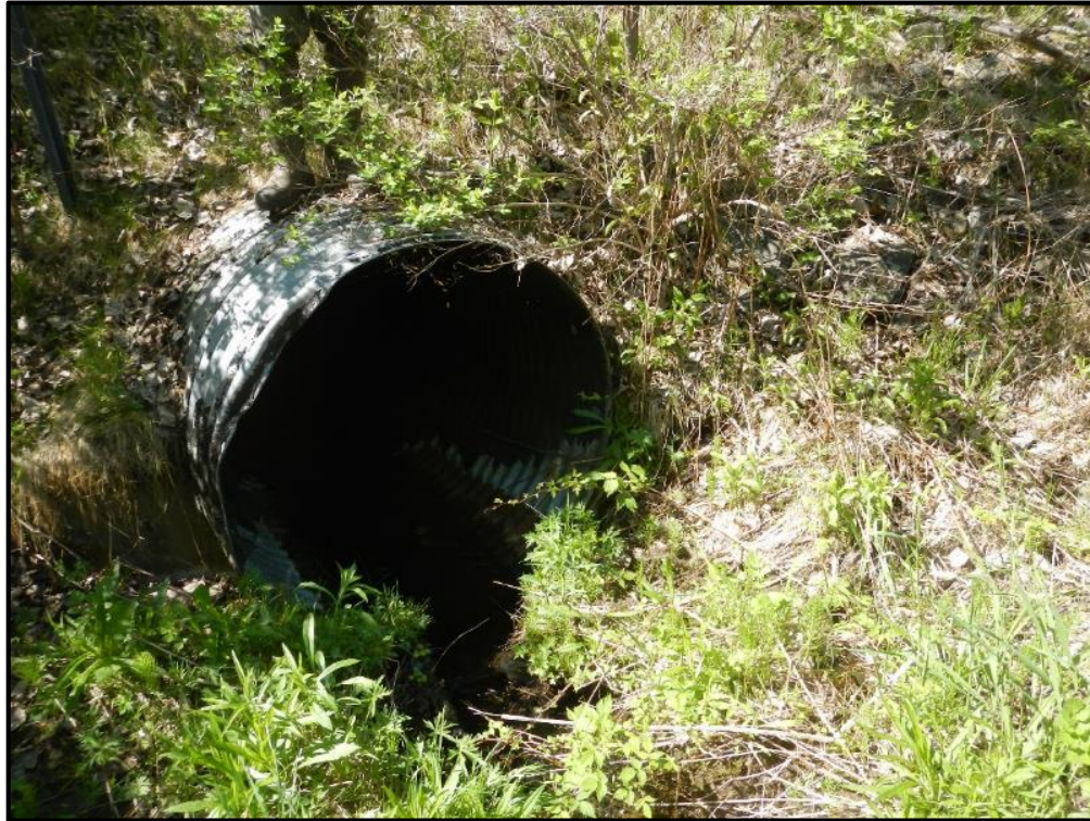
V-FH-S-17 Culvert Inlet
