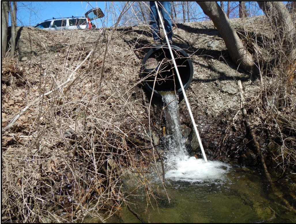
V-BE-AS-10 Culvert Outlet
