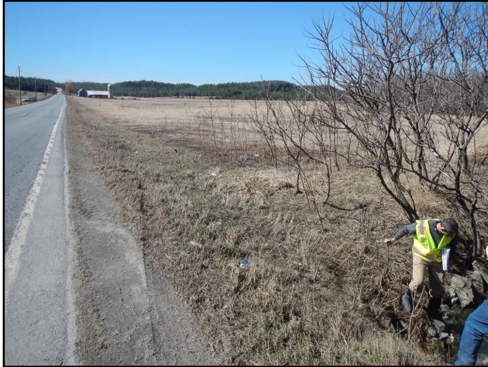
V-WH-S-4 Up Station Roadway
