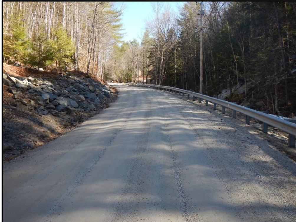
T-LU-S20 Up Station Roadway
