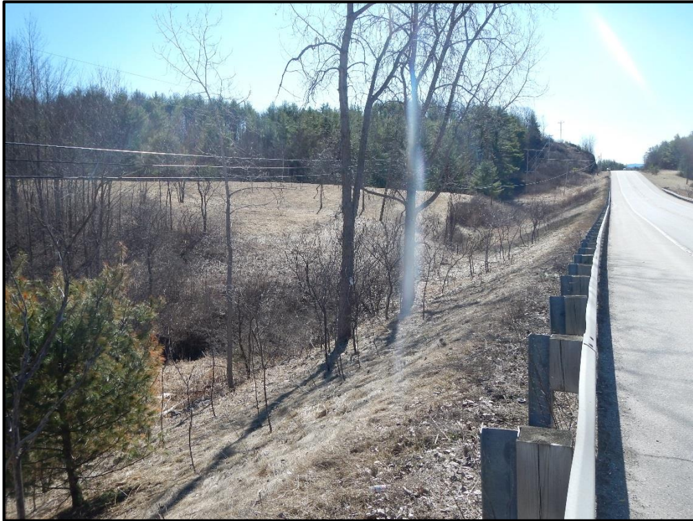
V-FH-S-17 Up Station Roadway
