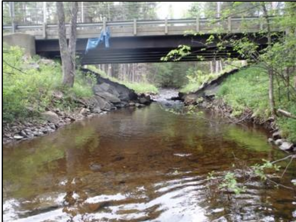
T-MH-S28 Channel Downstream of Bridge
