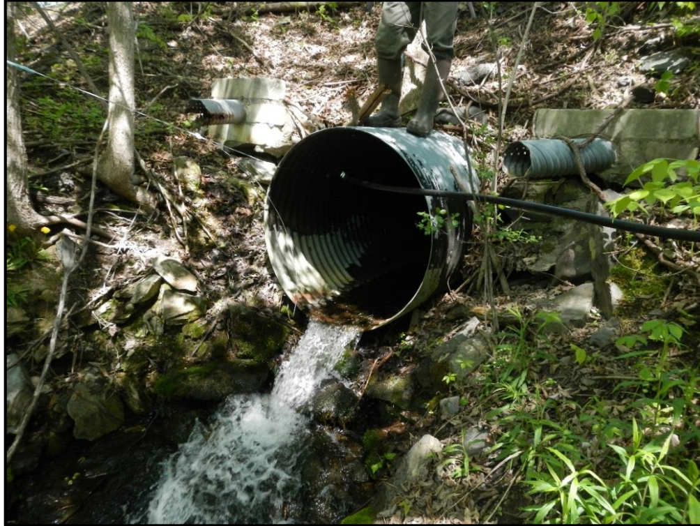
V-FH-S-25 Culvert Outlet
