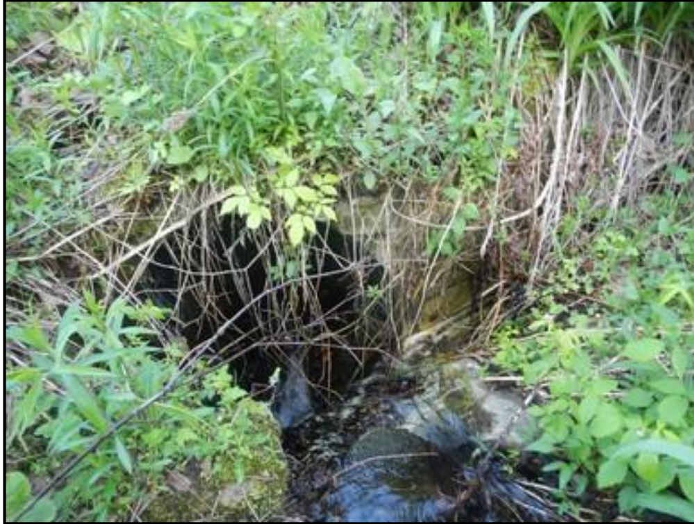
V-SH-S-16 Culvert Inlet; remnants of old headwall obstructing culvert inlet
