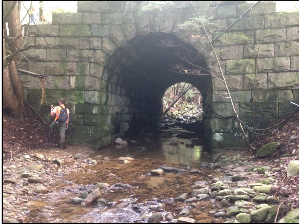
T-SH-S2 Culvert Outlet
