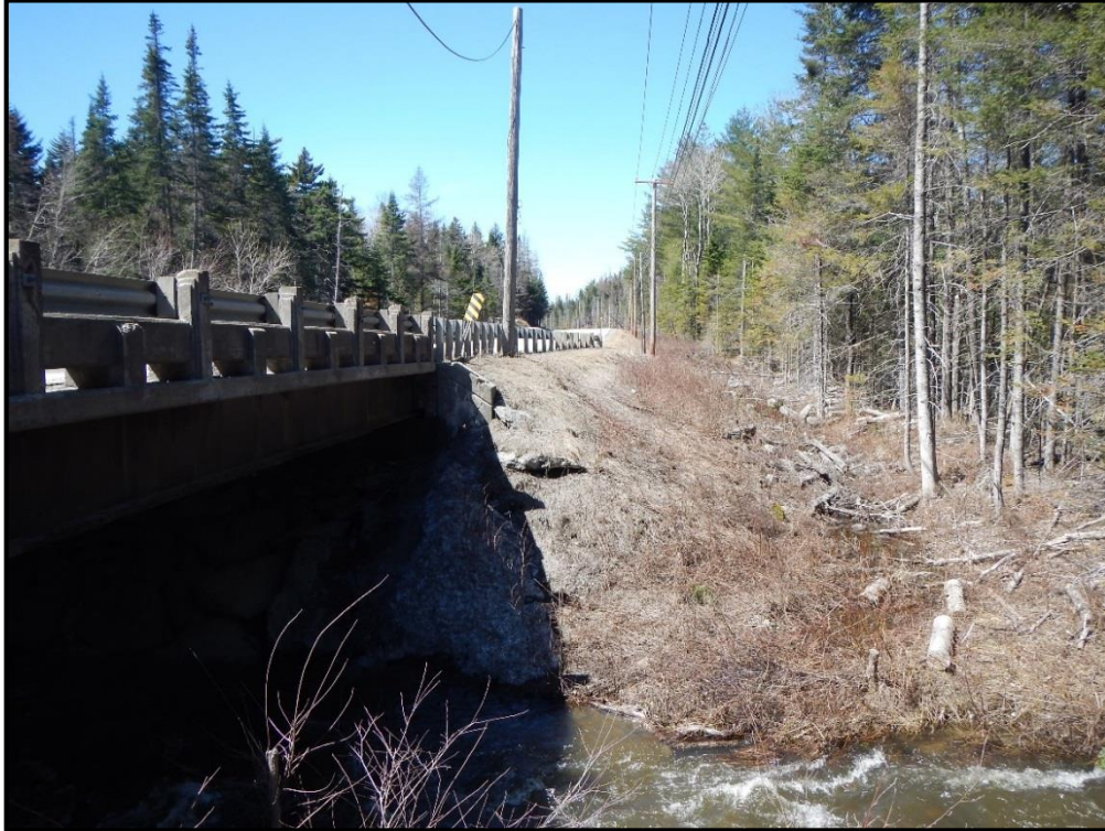
T-MH-S28 Upstream Bridge Abutment
