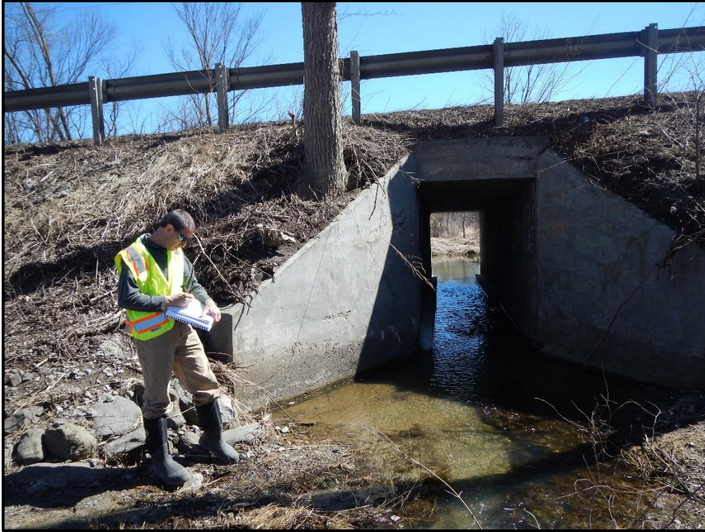
V-BE-S-102 Culvert Inlet
