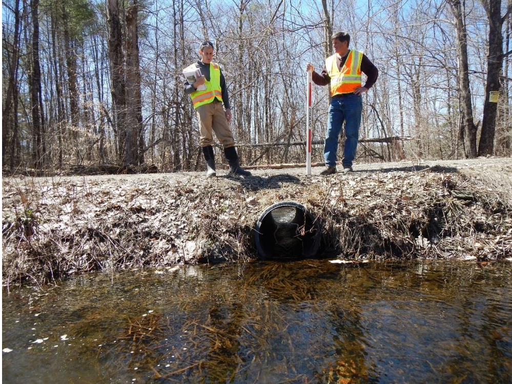
V-BE-S-8 Culvert Inlet
