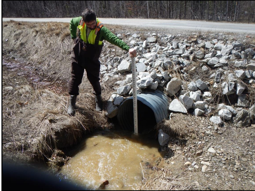
V-WA-S105 Culvert Inlet
