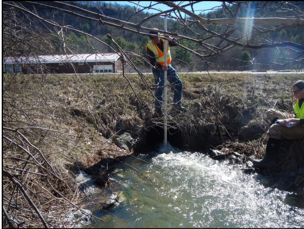
V-WH-S-4 Culvert Outlet
