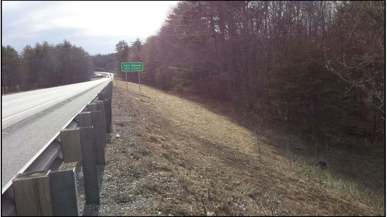
V-CN-S-101 Down Station Roadway
