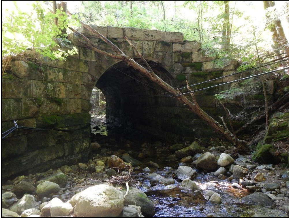
T-SH-S2 Culvert Inlet
