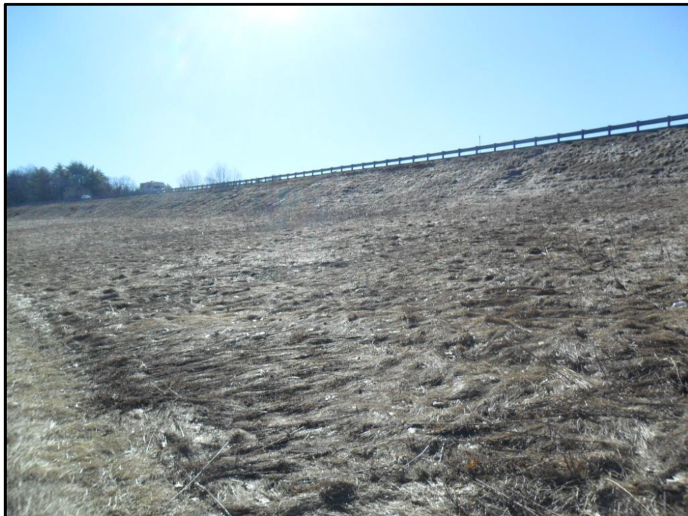
V-FH-S-10 Up Station Roadway
