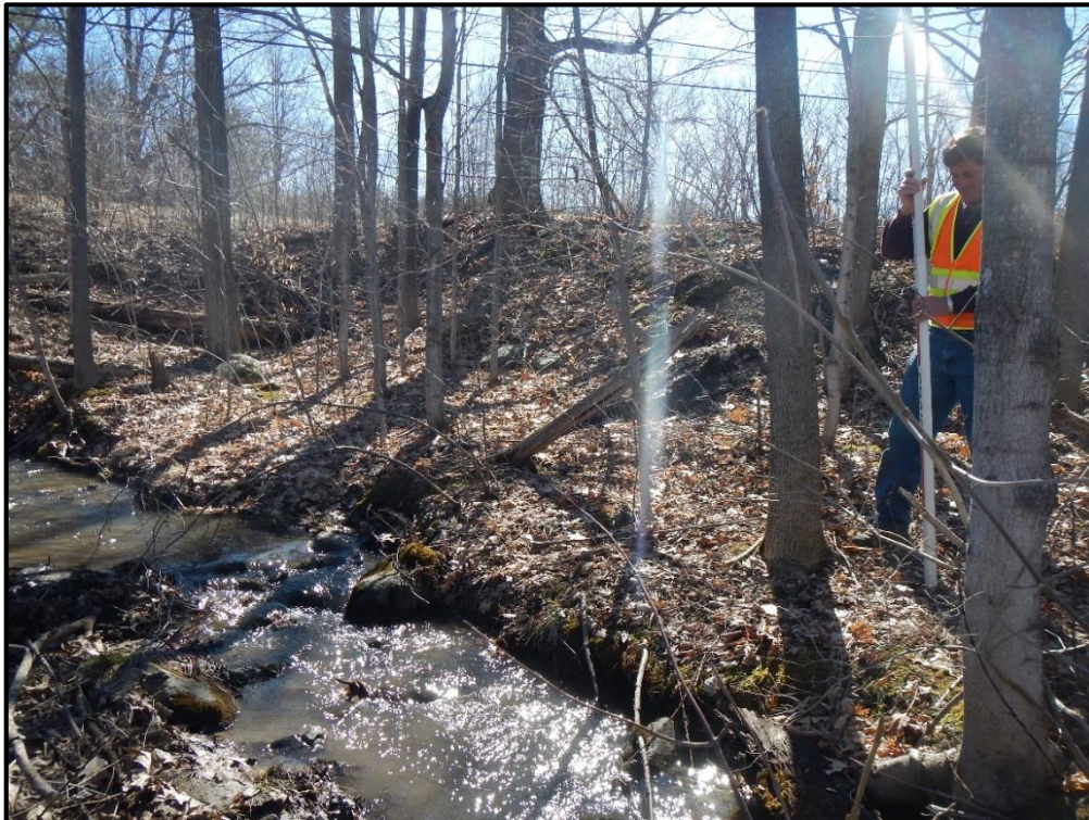
V-WH-S-2 View South of Downstream Culvert Outlet
