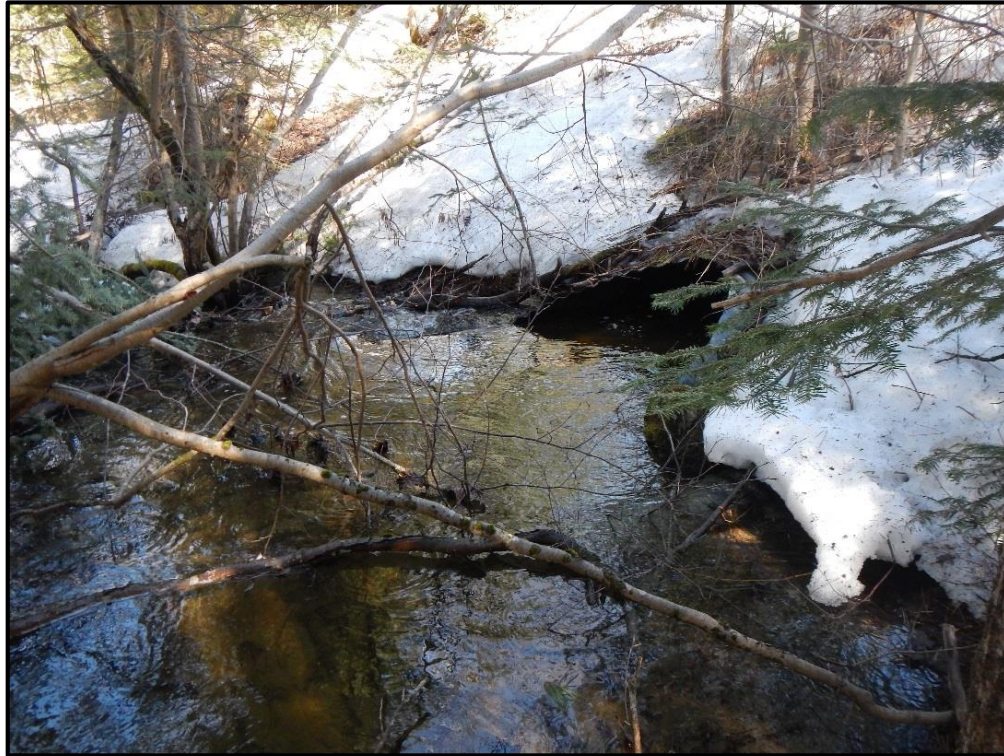
T-MH-AS-45 Downstream Culvert
