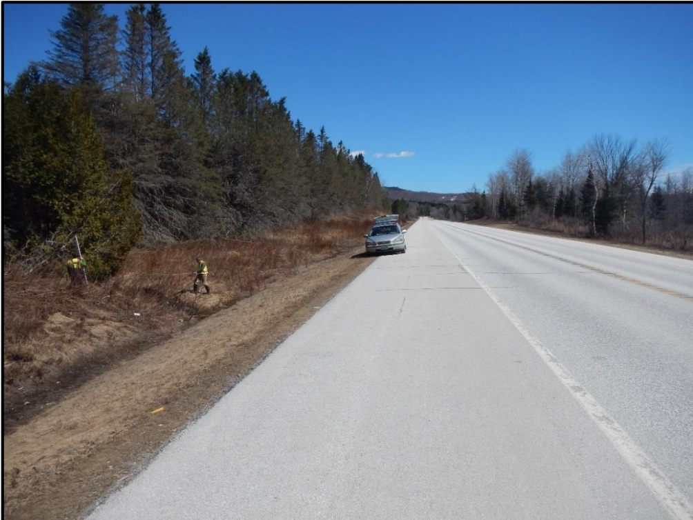
T-MH-AS-23 Up Station Roadway
