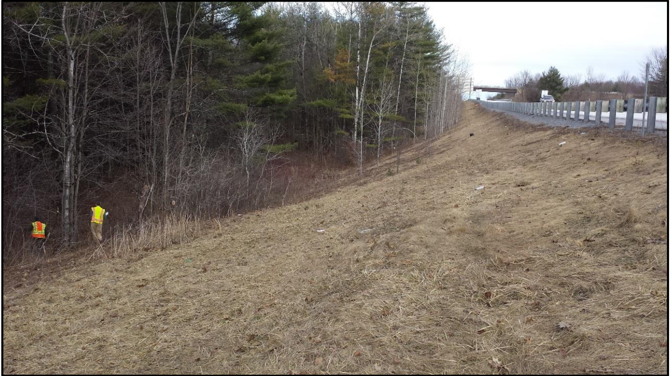
V-FH-S-5 Up Station Roadway
