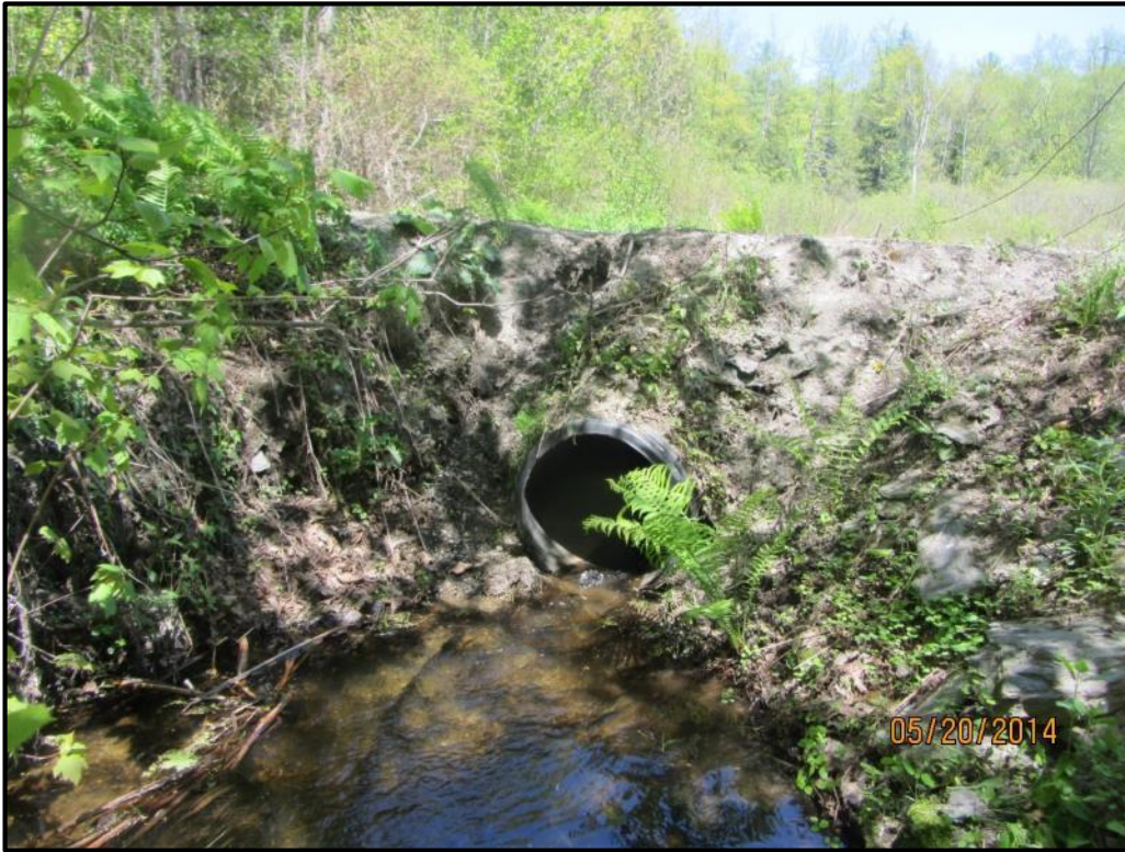
V-BE-S-8 Culvert Outlet
