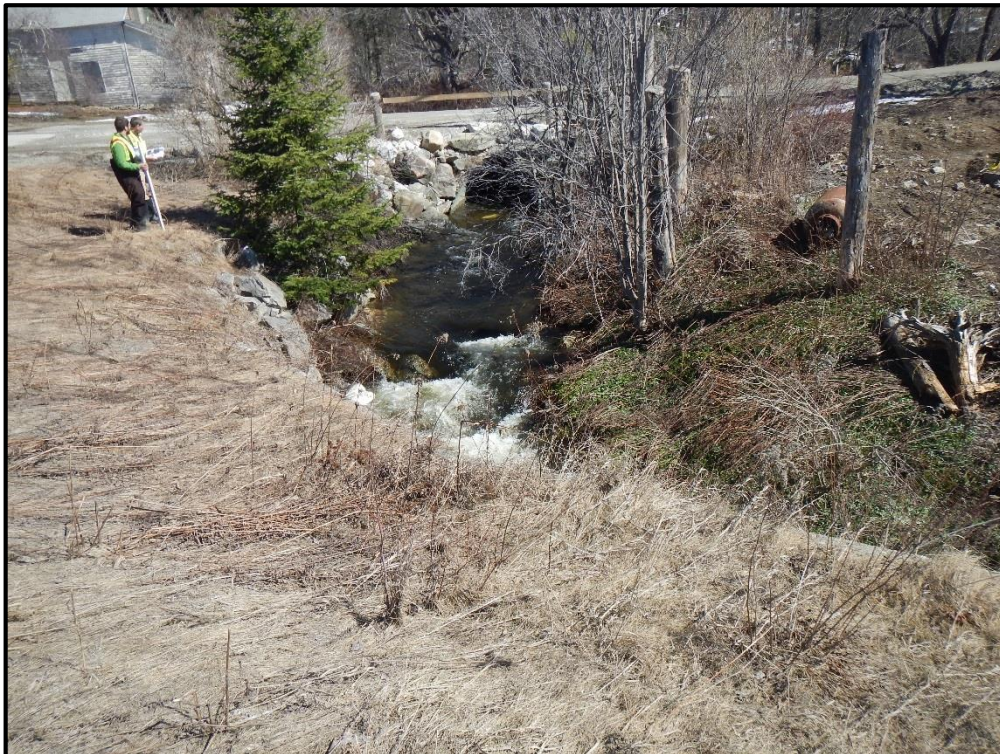
T-MH-S-14 Upstream Channel
