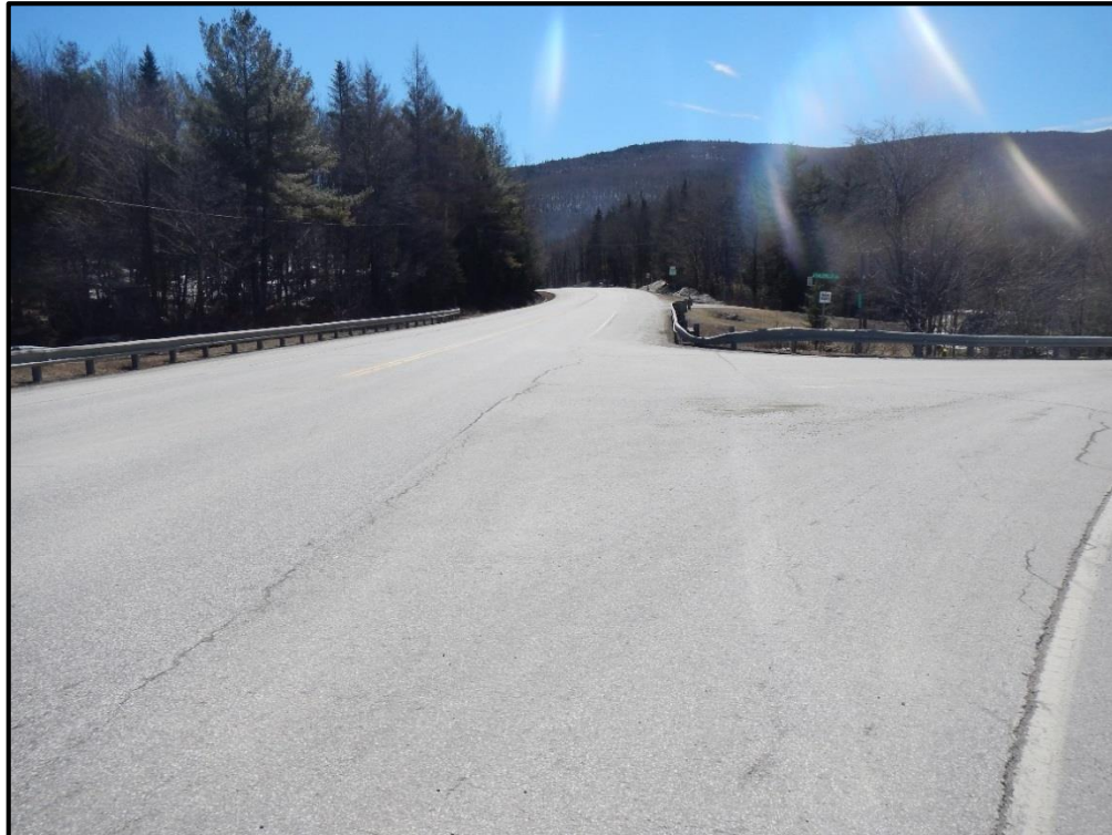
T-MH-S14 Up Station Roadway
