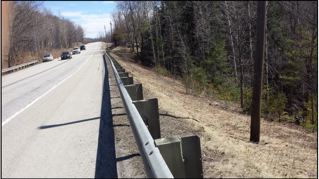
V-SH-S-14 Up Station Roadway
