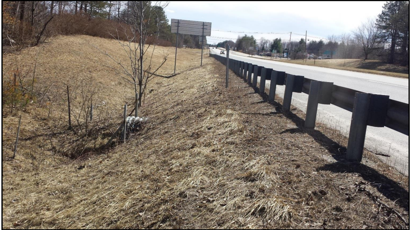
T-CL-S4 Up Station Roadway; top of cattle pass visible at ditch line
