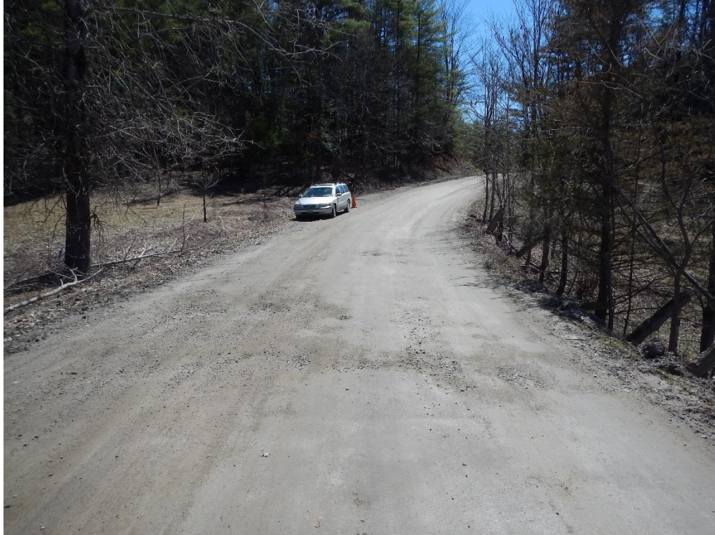
V-BE-AS-3 Up Station Roadway
