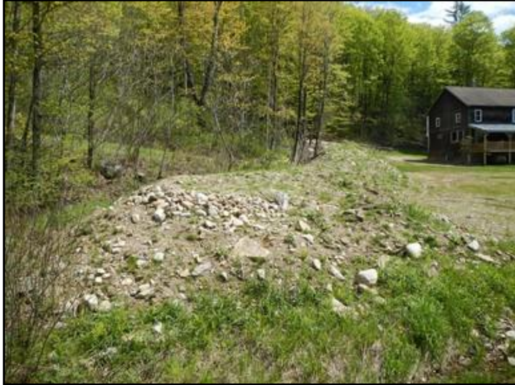
V-WA-S105 Flood Berm Adjacent To Upstream Channel
