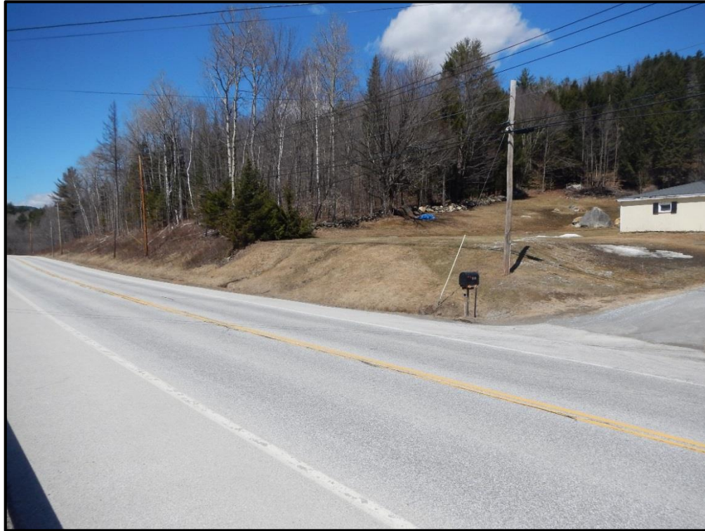
T-MH-S37 Down Station Roadway
