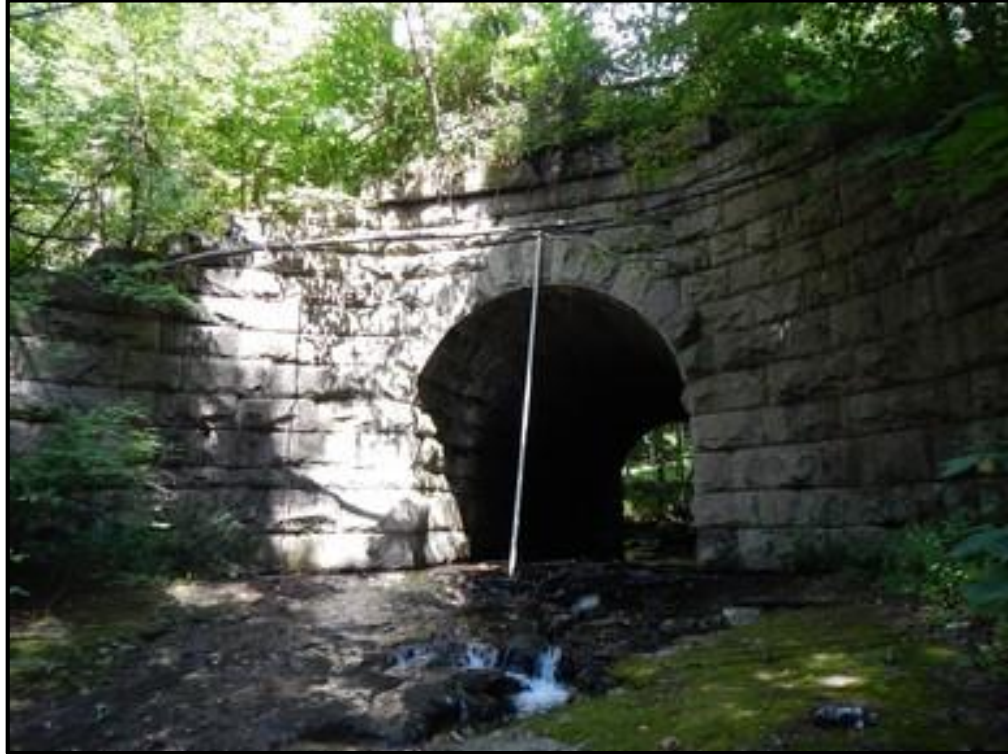
T-SH-S3 Culvert Outlet
