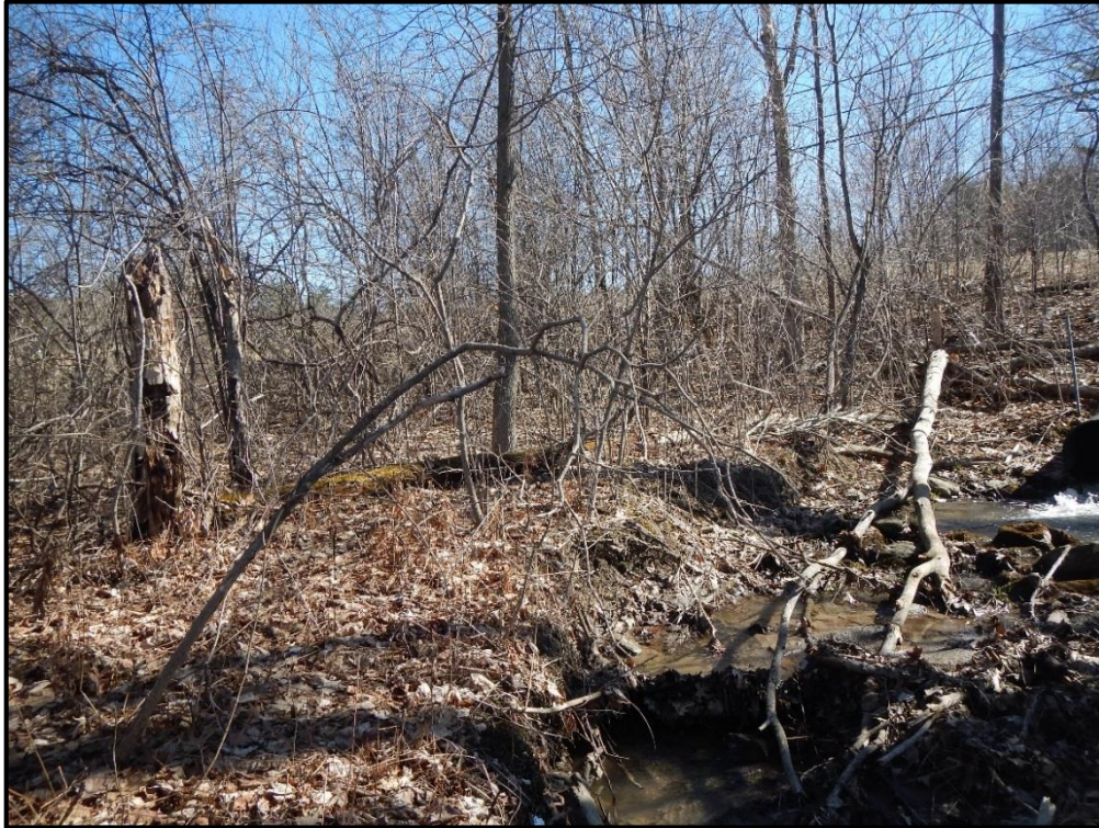
V-WH-S-2 View North of Downstream Culvert Outlet
