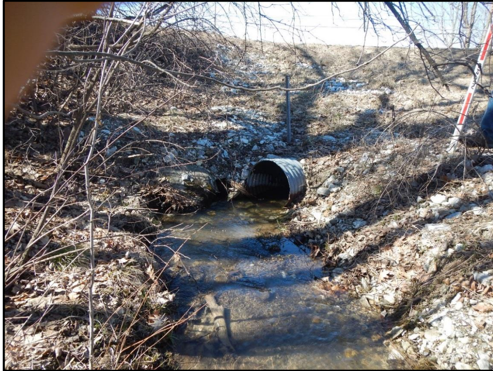
V-WH-S-2 Culvert Inlet
