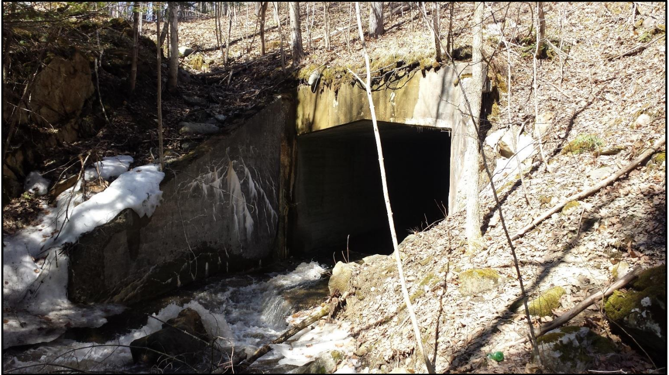
V-SH-S-14 Culvert Outlet
