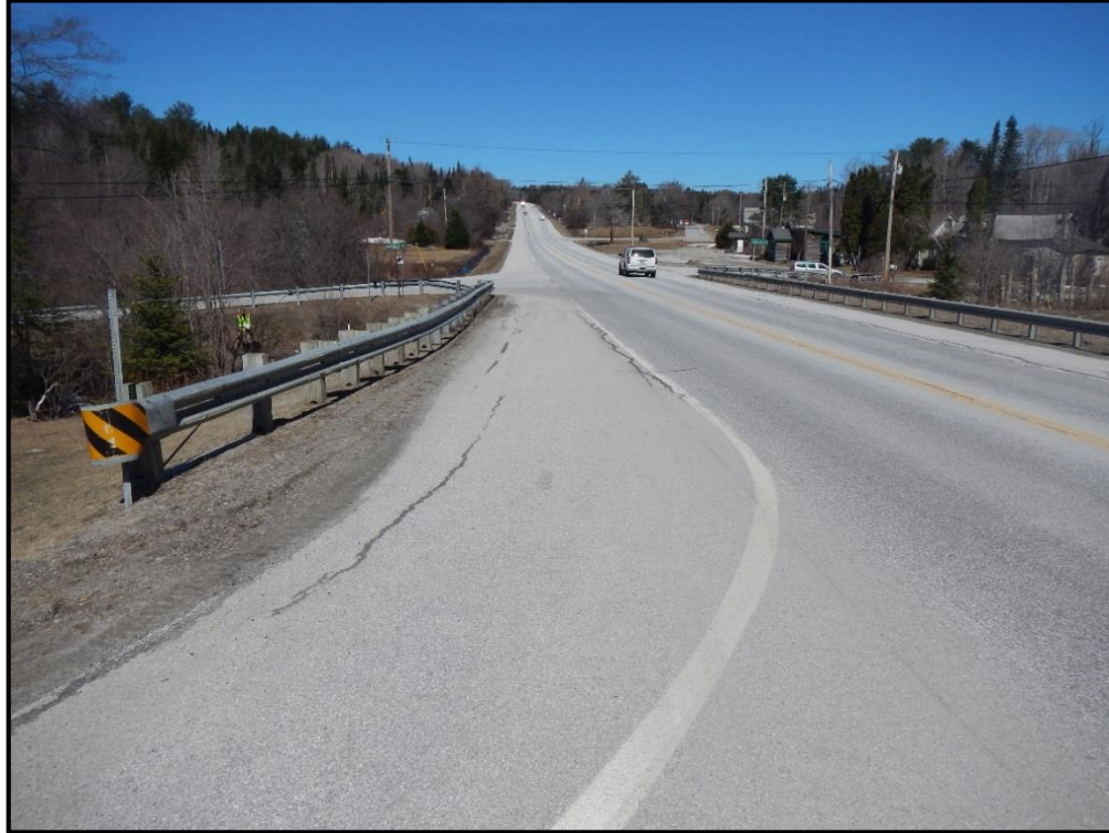
T-MH-S14 Down Station Roadway
