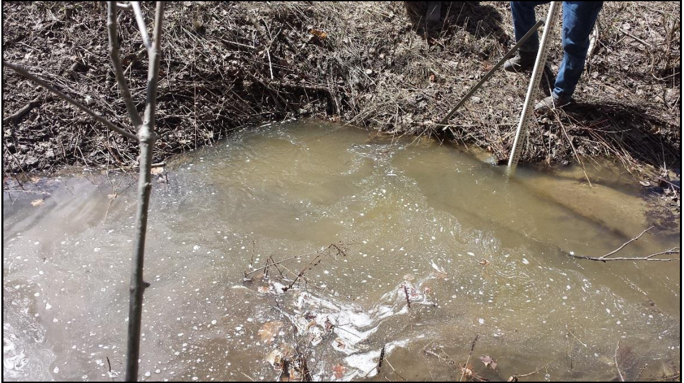
V-WA-S106 Culvert Inlet (partially clogged and submerged)
