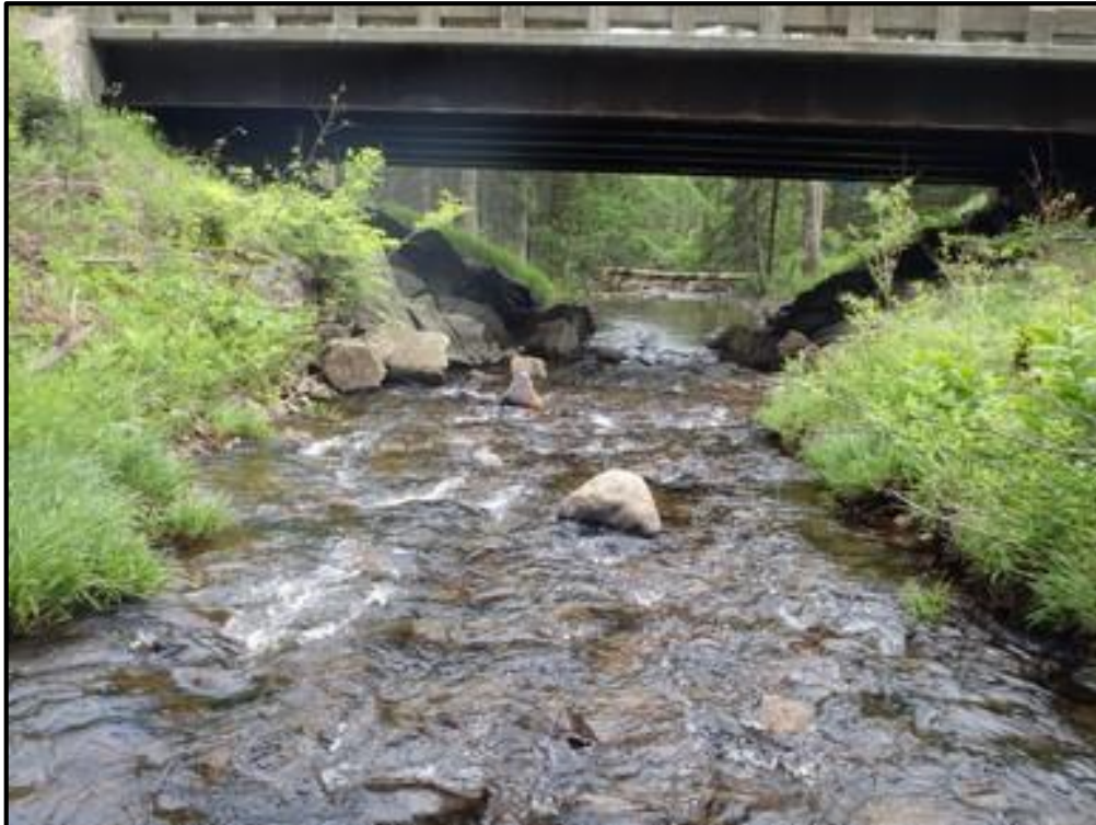
T-MH-S28 Channel Upstream of Bridge
