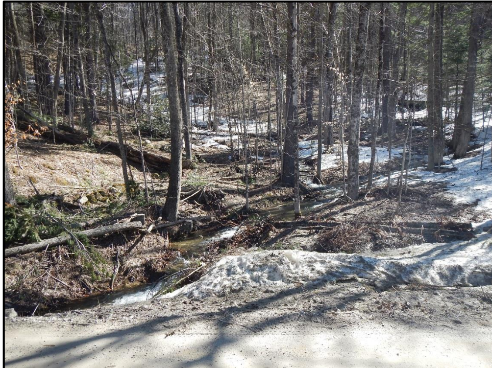
T-LU-S21 Upstream Channel
