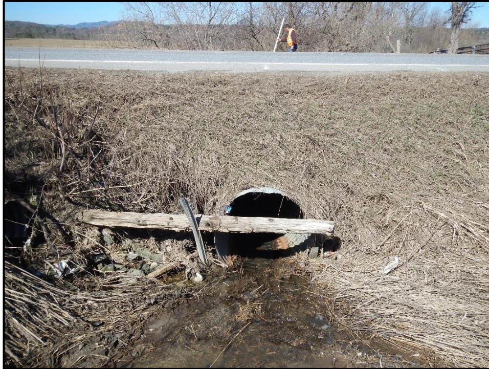
V-BE-S-109 Culvert Inlet
