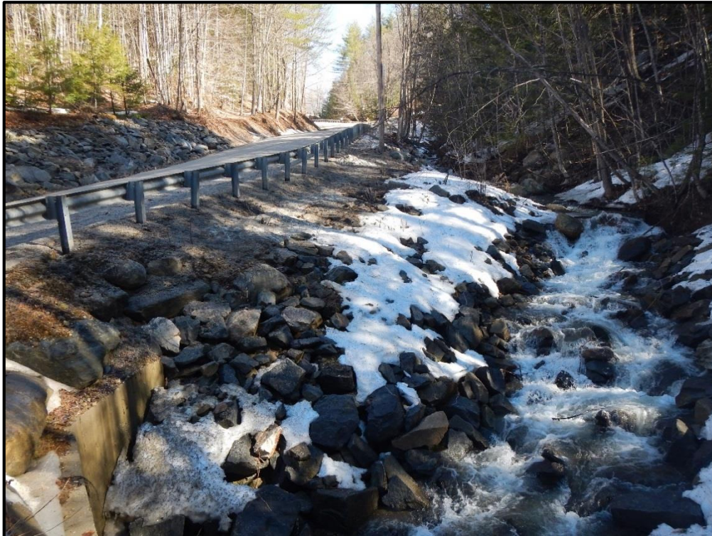
T-LU-S20 Upstream Channel
