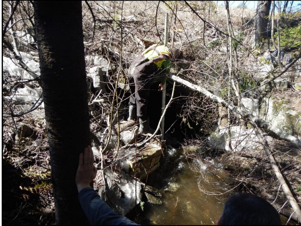
T-MH-AS-20 Culvert Inlet
