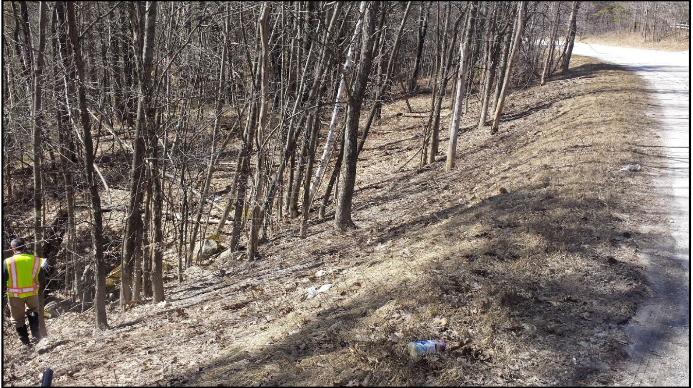
V-SH-S-16 Up Station Roadway
