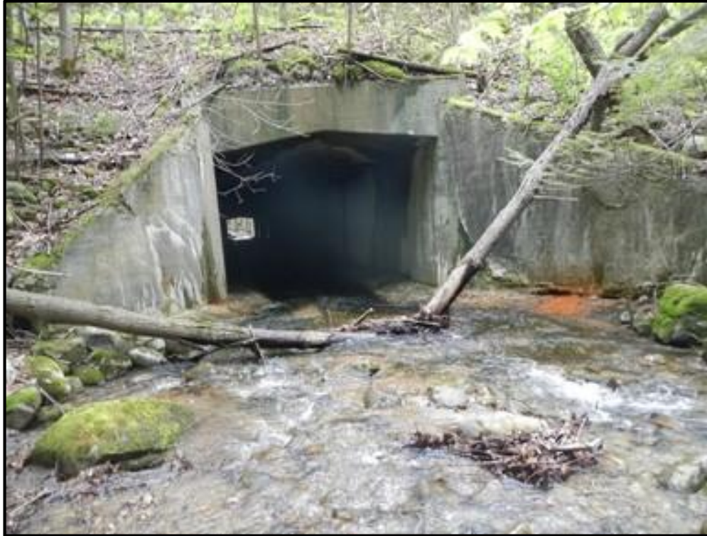
V-SH-S-14 Culvert Inlet
