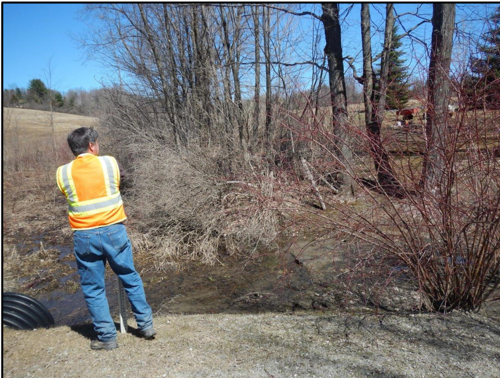
V-BE-AS-10 Culvert Inlet / Upstream Wetland (V-BE-AS-17)
