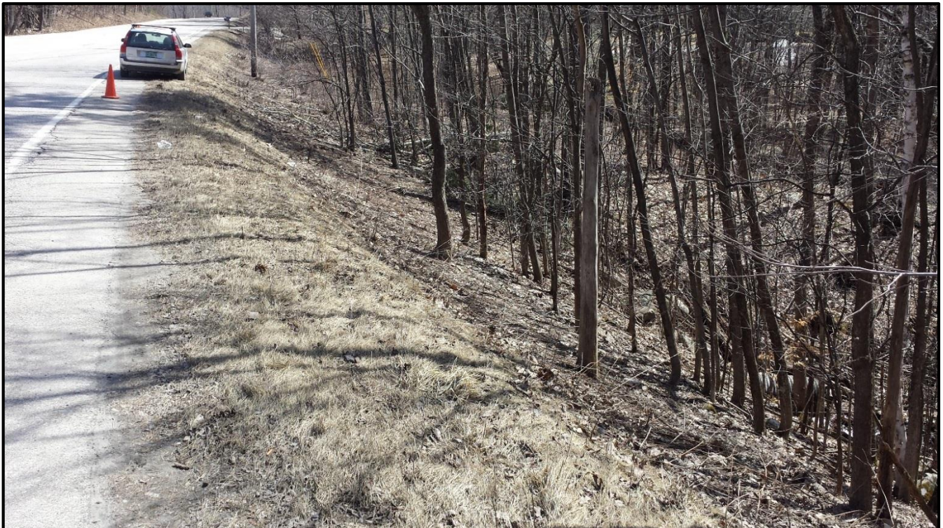
V-SH-S-16 Down Station Roadway
