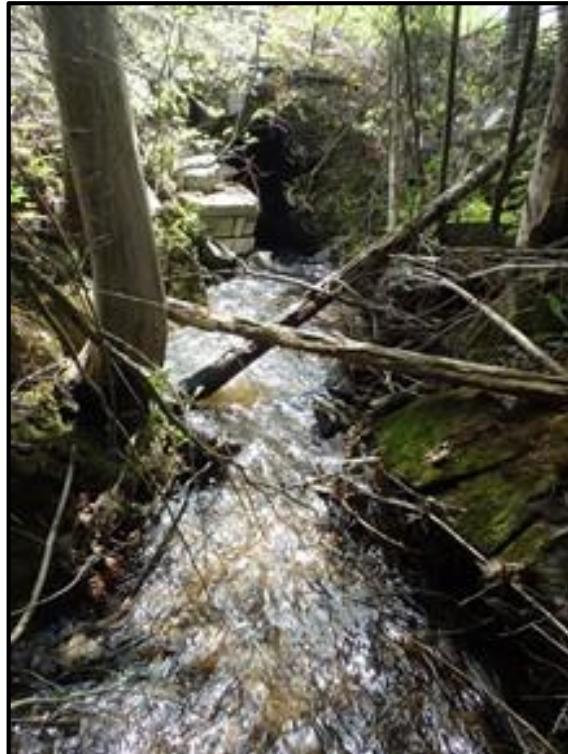
T-MH-AS-20 Upstream Channel
