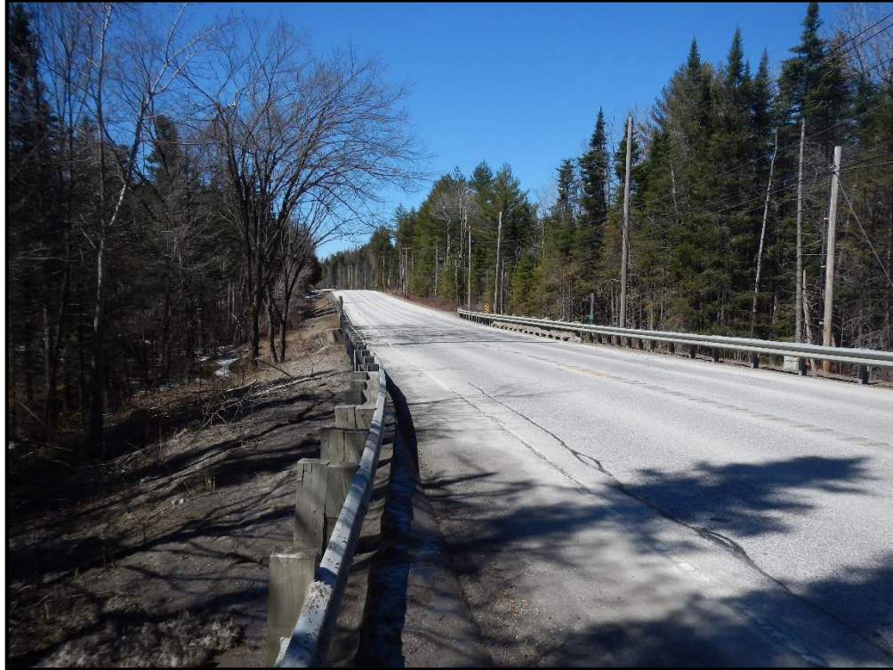
T-MH-S28 Downstream Bridge Abutment
