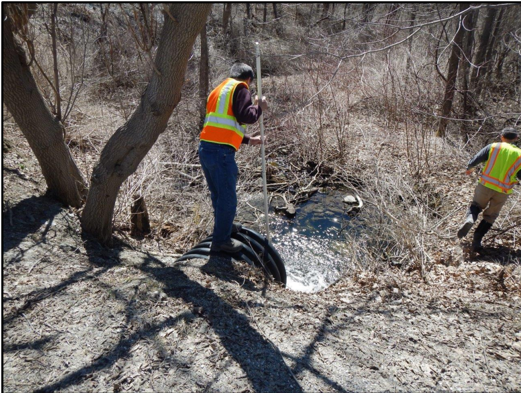
V-BE-AS-10 Culvert Outlet Downstream
