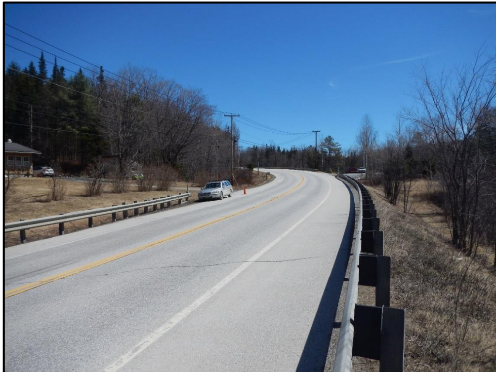
T-MH-S37 Up Station Roadway
