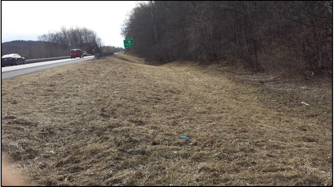
V-CN-S-4 Down Station Roadway
