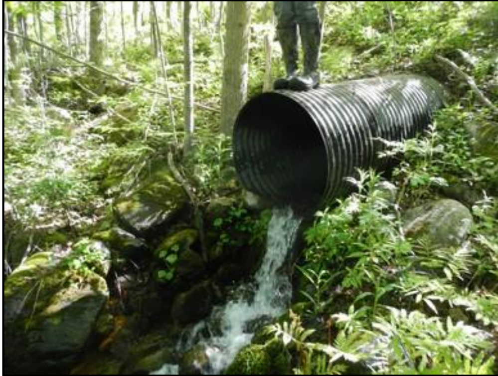
V-SH-S-16 Culvert Outlet
