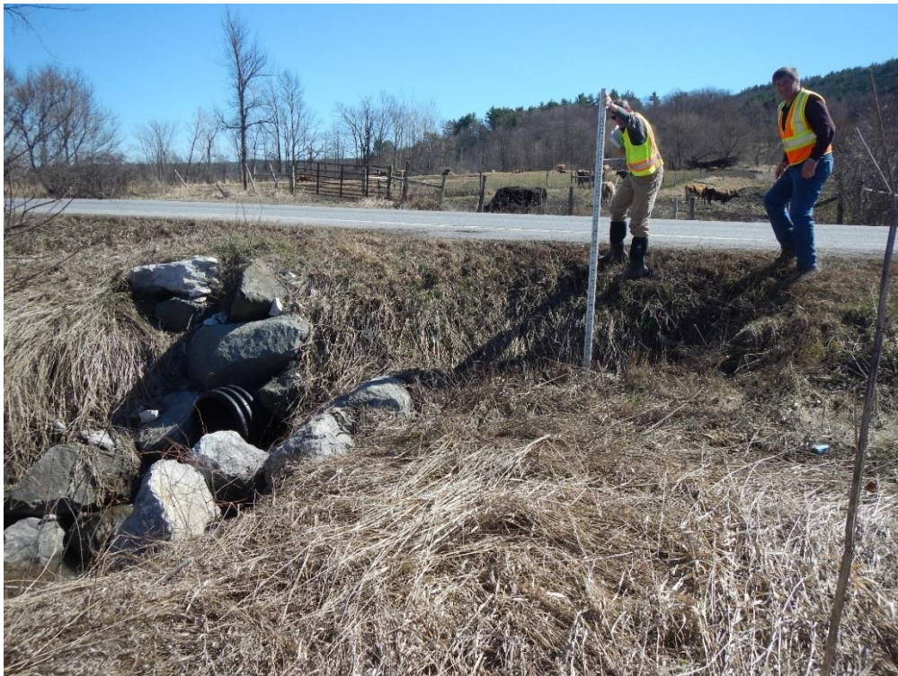
V-BE-S-109 Gully within ROW, south of culvert crossing
