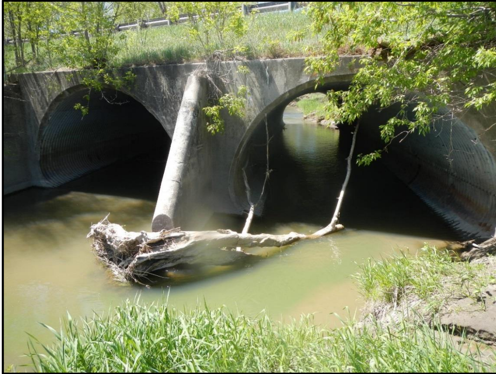
V-BE-S-106 double culvert inlet
