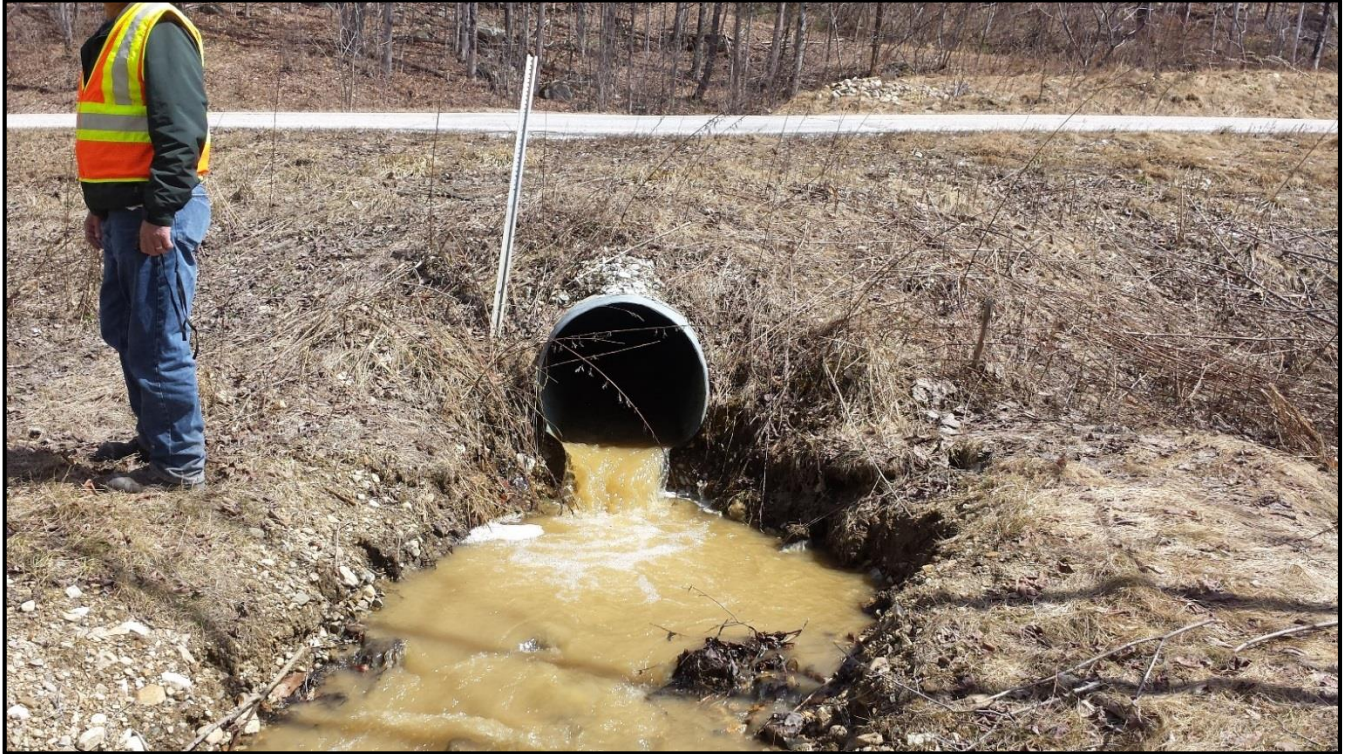
V-WA-S106 Culvert Outlet
