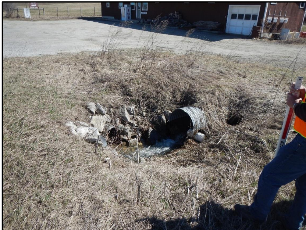
V-WH-S-4 Upstream Culverts (Northeast)
