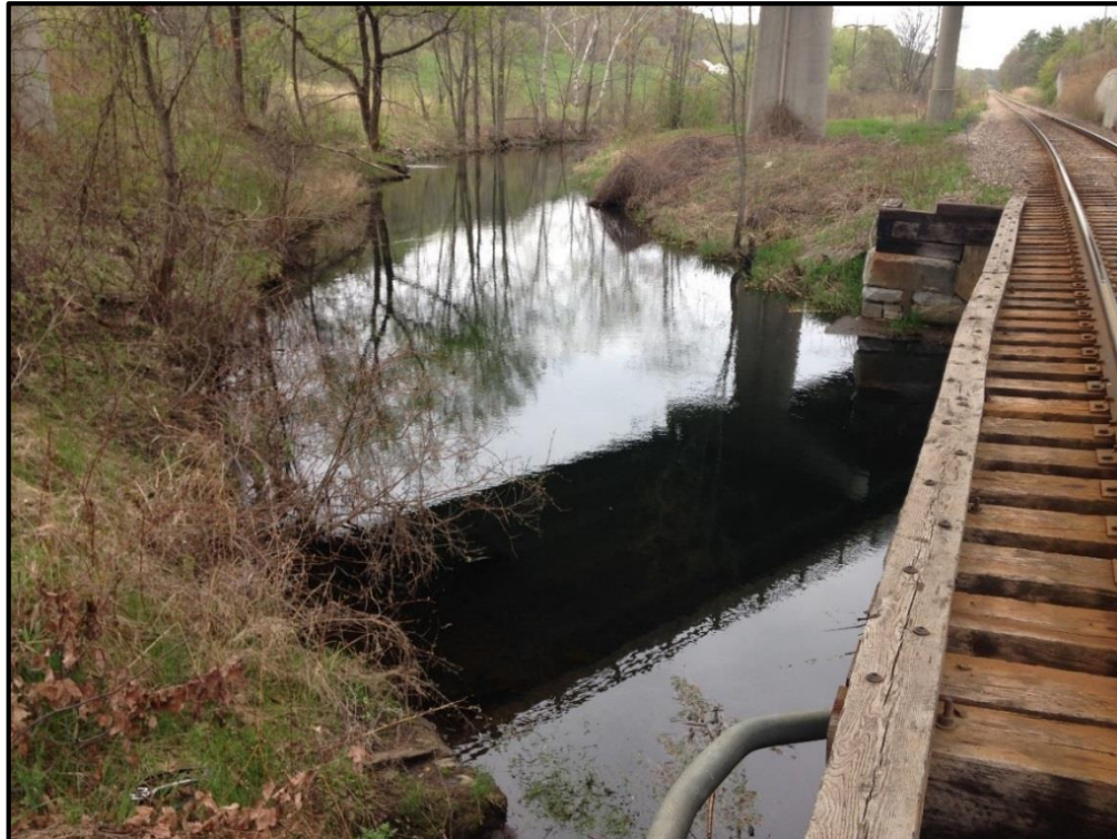
T-WR-S29 Upstream Channel
