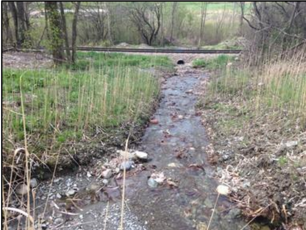
T-WR-S34 Downstream Channel
