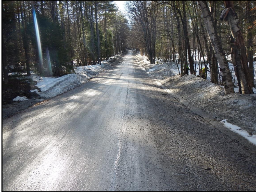
T-LU-S12 Up Station Roadway
