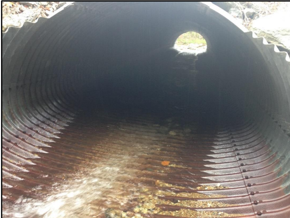
T-LU-S4 Culvert Interior
