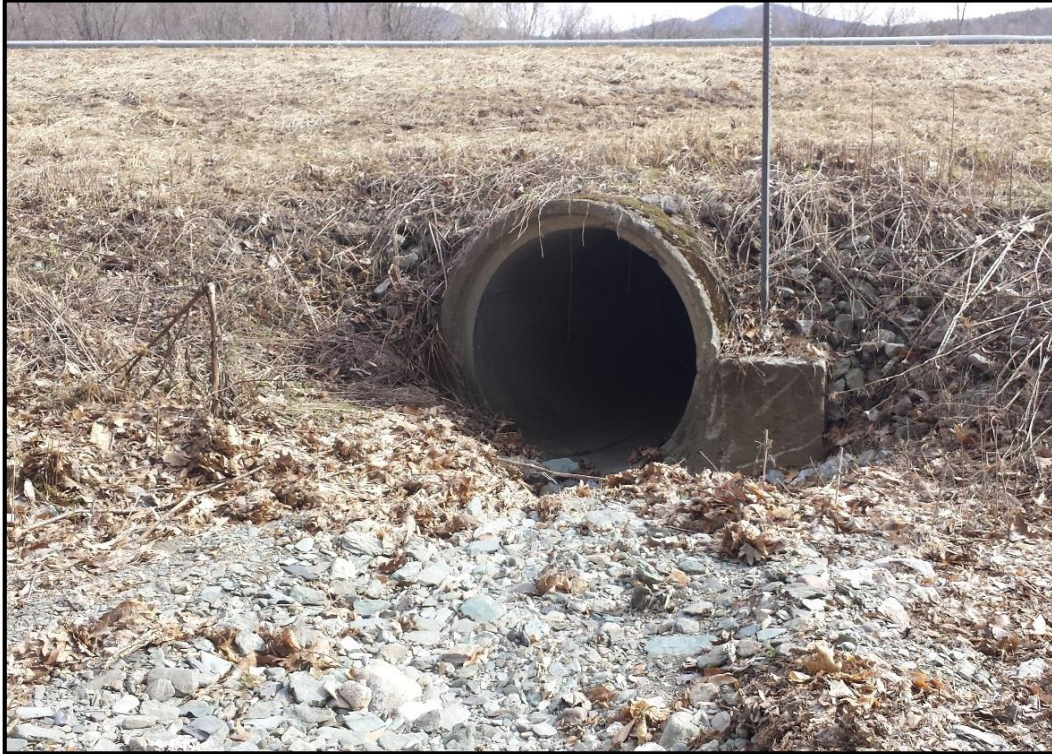
V-CN-S-4 Culvert Inlet
