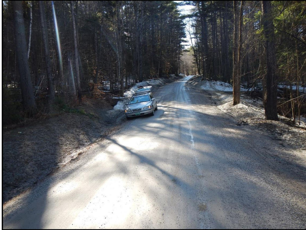
T-LU-S15 Up Station Roadway
