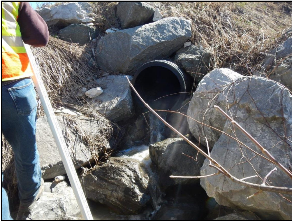
V-BE-S-109 Culvert Outlet
