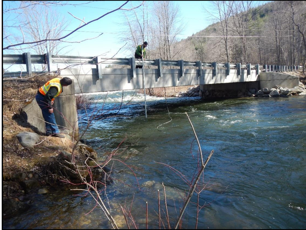
T-LU-S1 Downstream Face of Bridge
