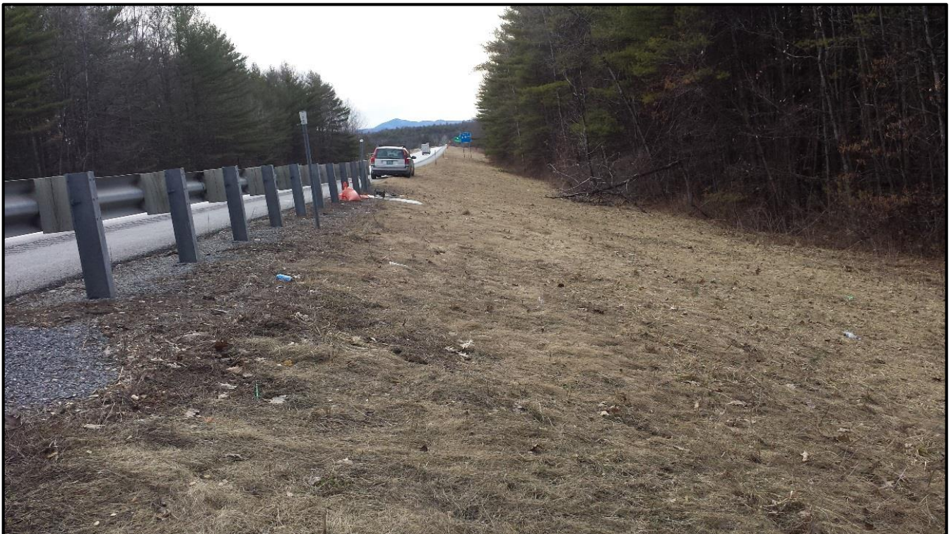
V-FH-S-5 Down Station Roadway
