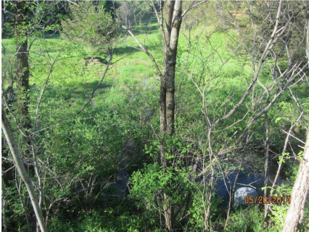
V-BE-AS-3 Culvert Outlet / Downstream Wetland (V-BE-AW-4)
