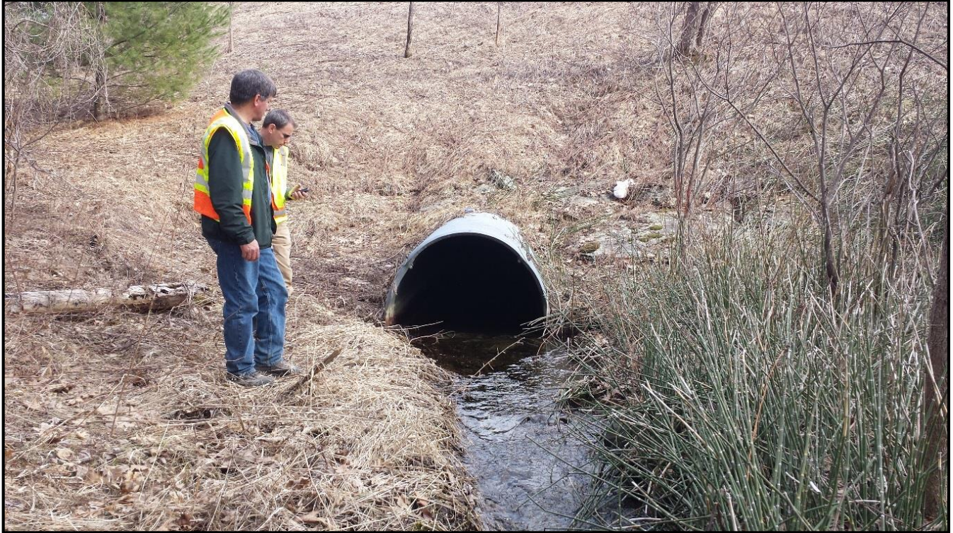
V-CN-S-101 Culvert Outlet
