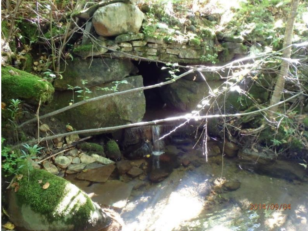
T-SH-S7 Culvert Outlet
