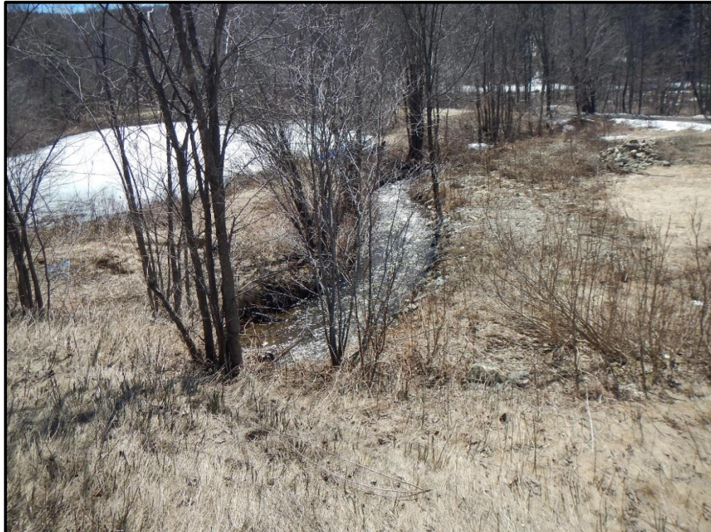
T-MH-S37 Downstream Channel
