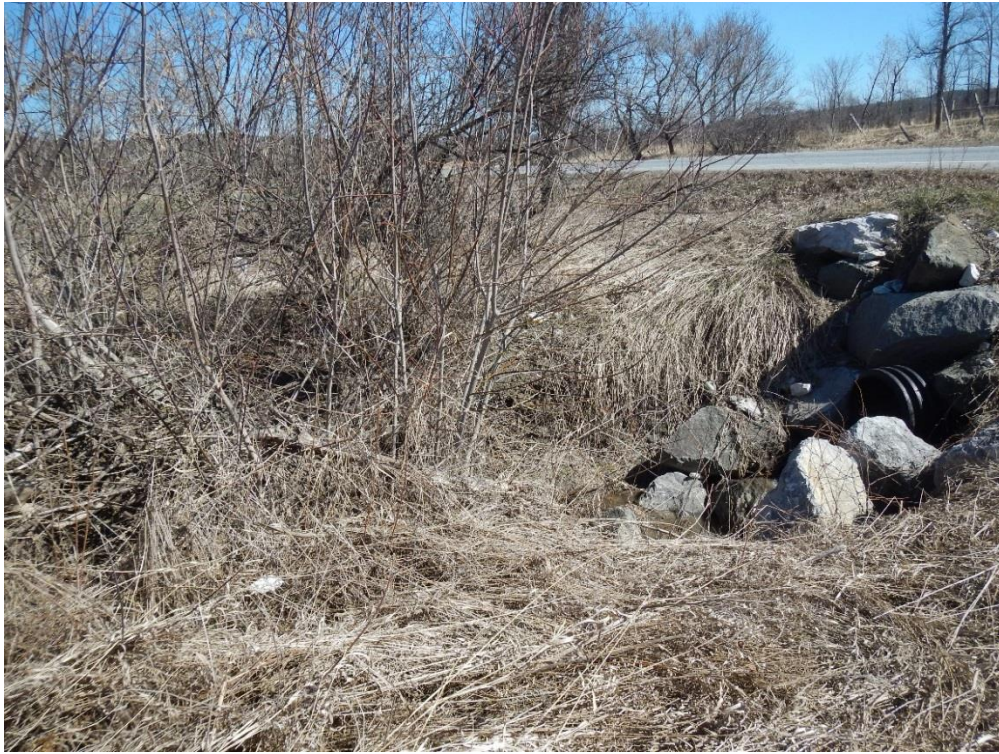
V-BE-S-109 Down Station Roadway
