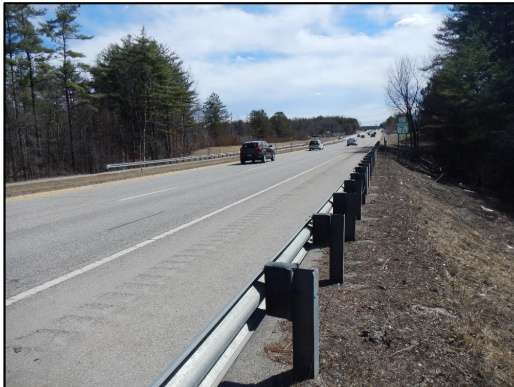
T-CL-S4 Down Station Roadway
