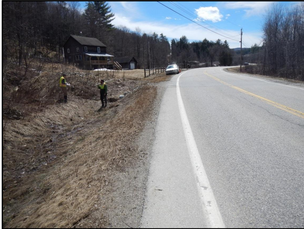
V-WA-S105 Down Station Roadway
