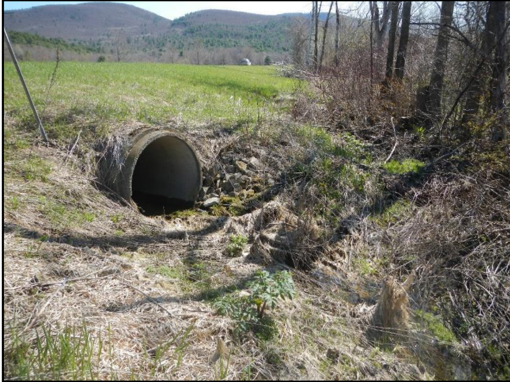
V-CN-S-4 Culvert Outlet
