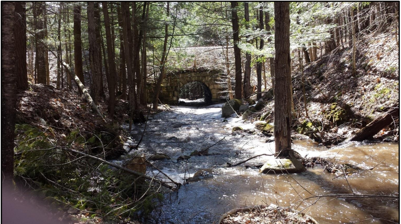
V-SH-S-14 Downstream Channel
