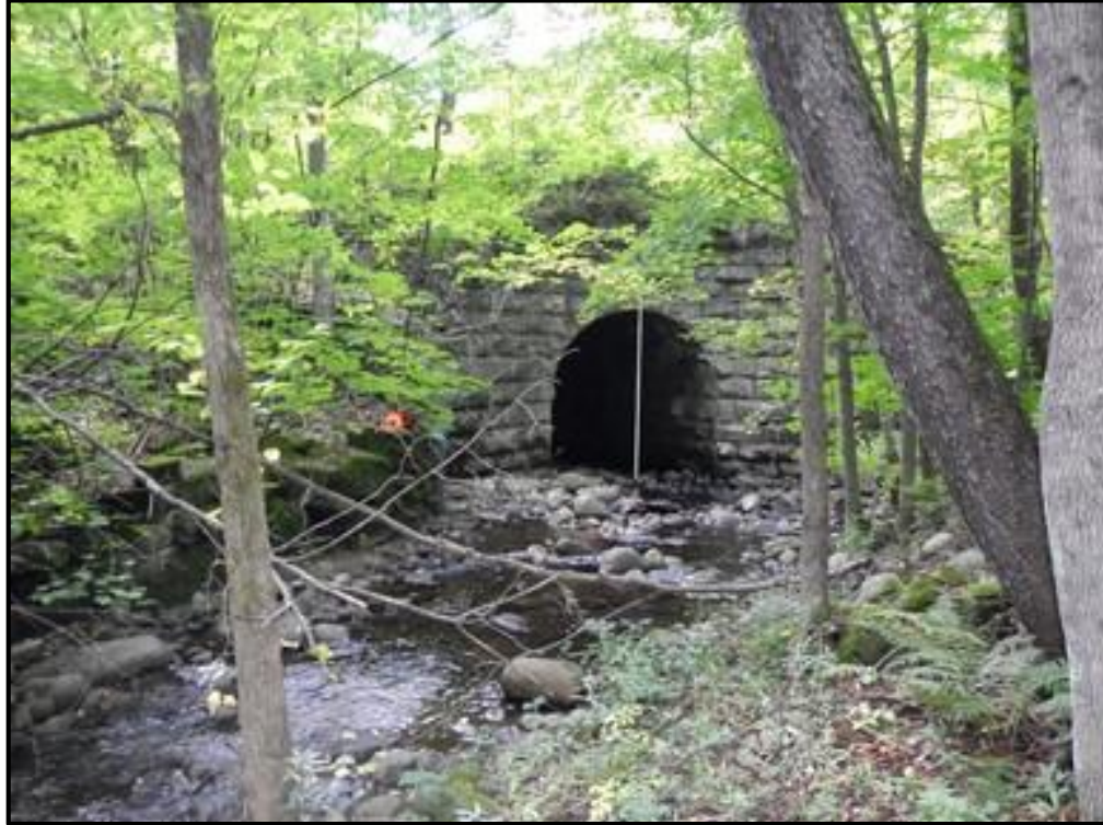
T-SH-S3 Culvert Inlet
