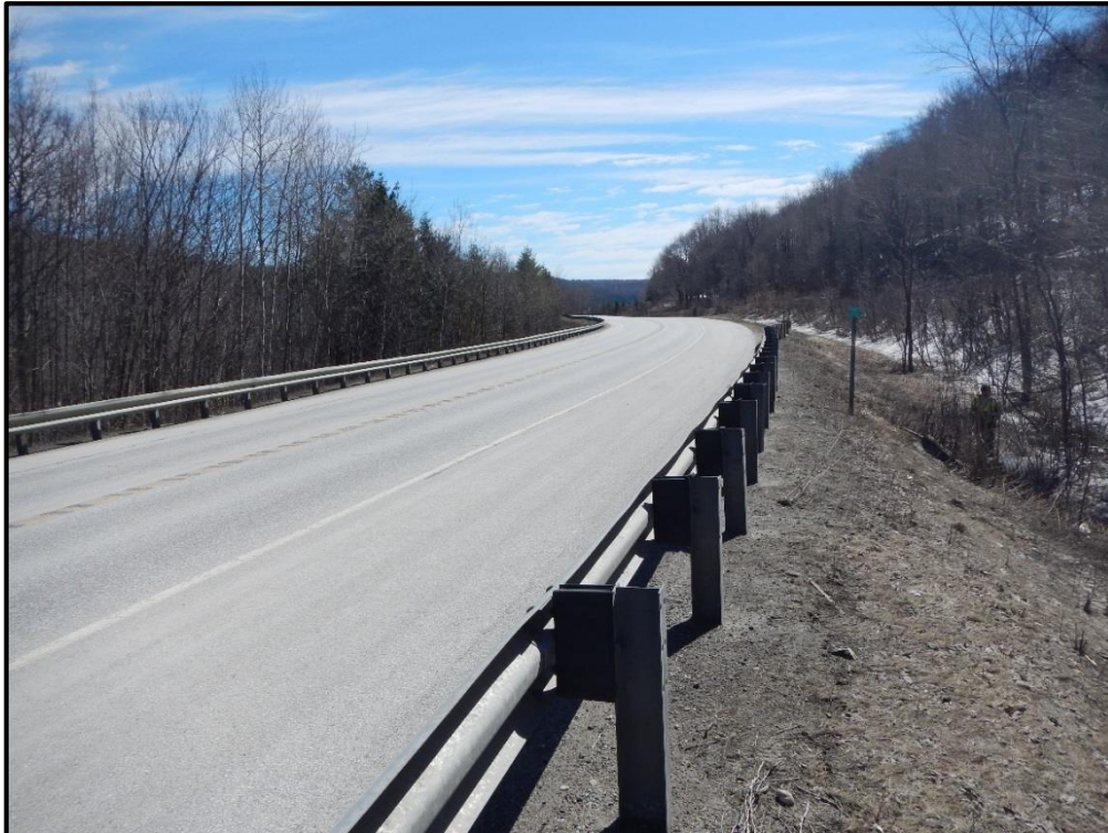
T-MH-S1 Up Station Roadway
