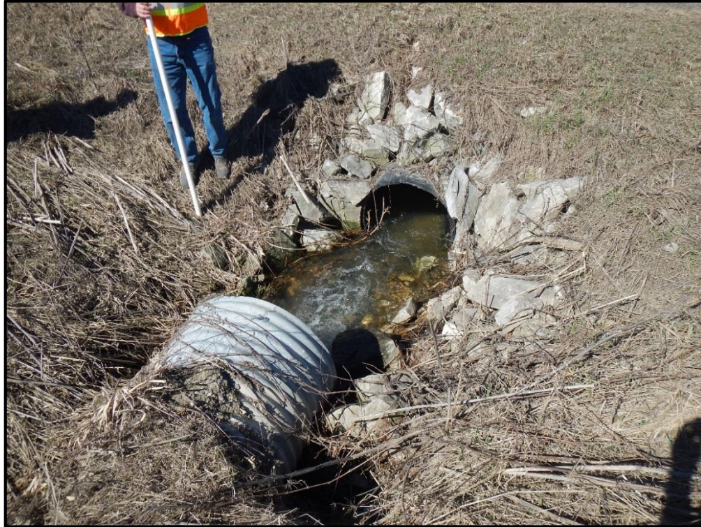
V-WH-S-4 Culvert Inlet
