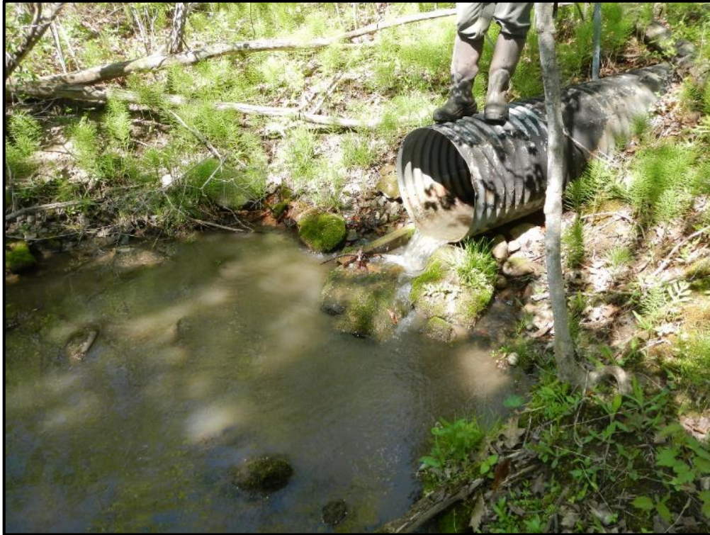
V-WH-S-2 Culvert Outlet
