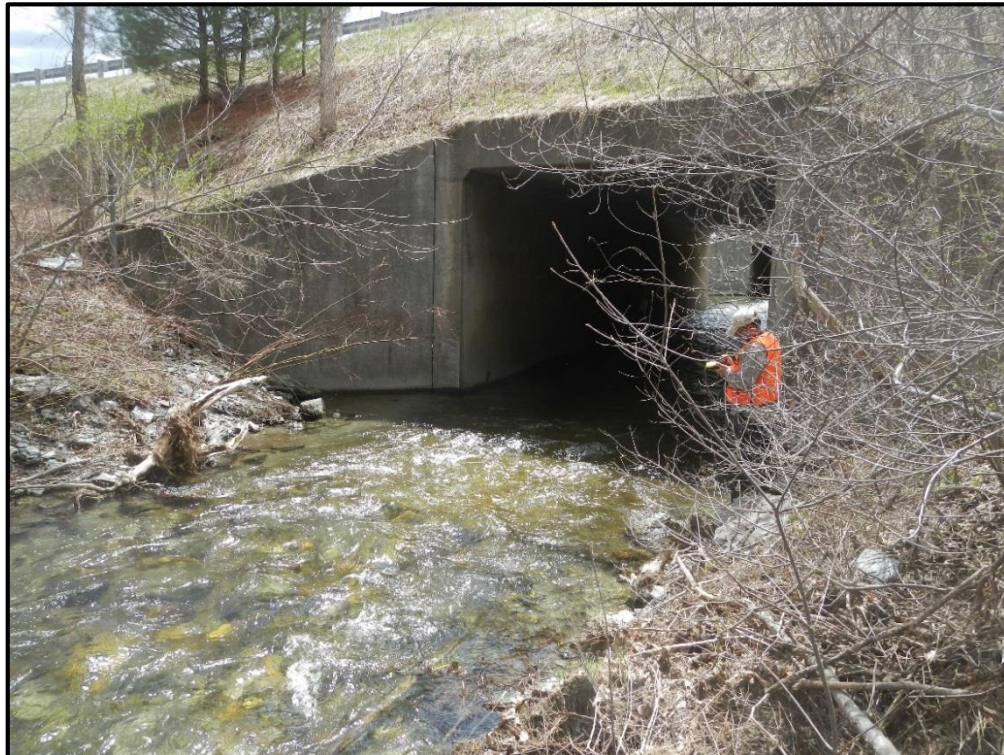
V-CN-S-8 Culvert Inlet
