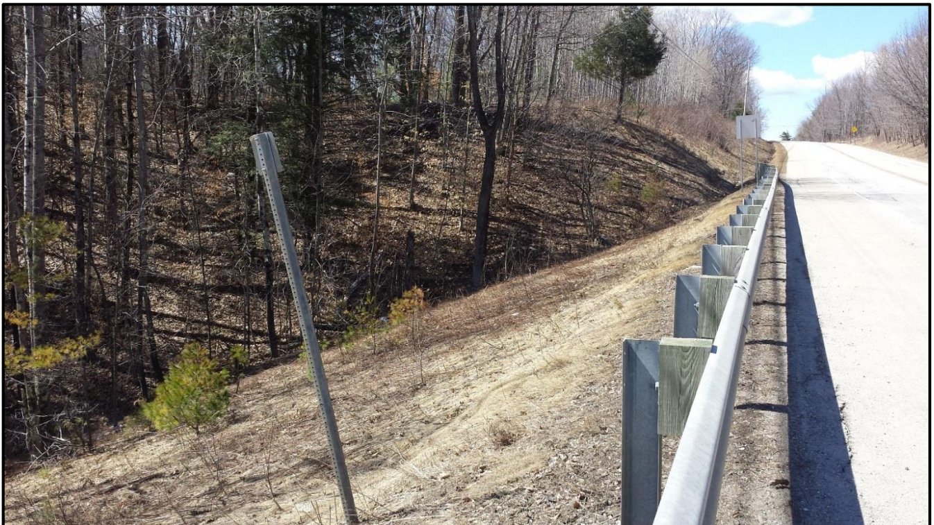
V-SH-S-14 Down Station Roadway
