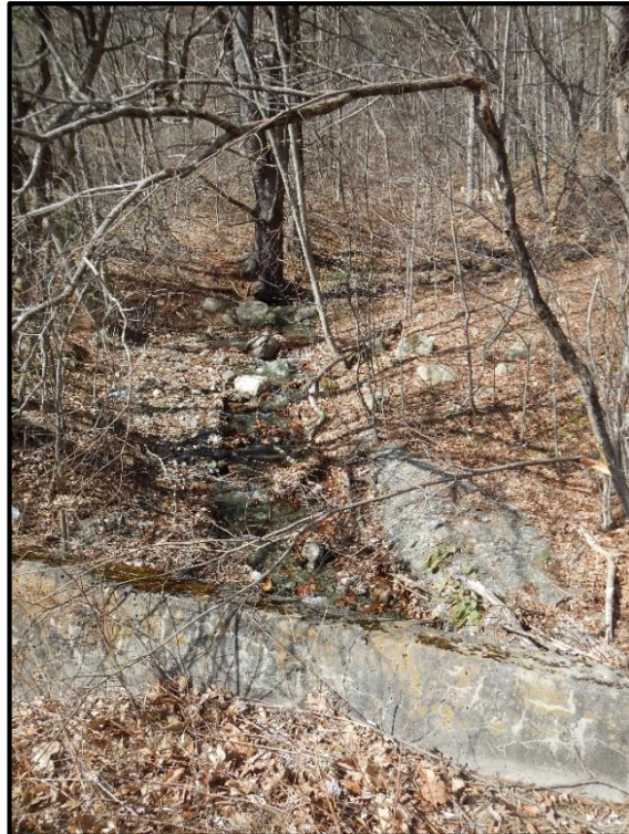
T-WR-S34 Upstream Channel
