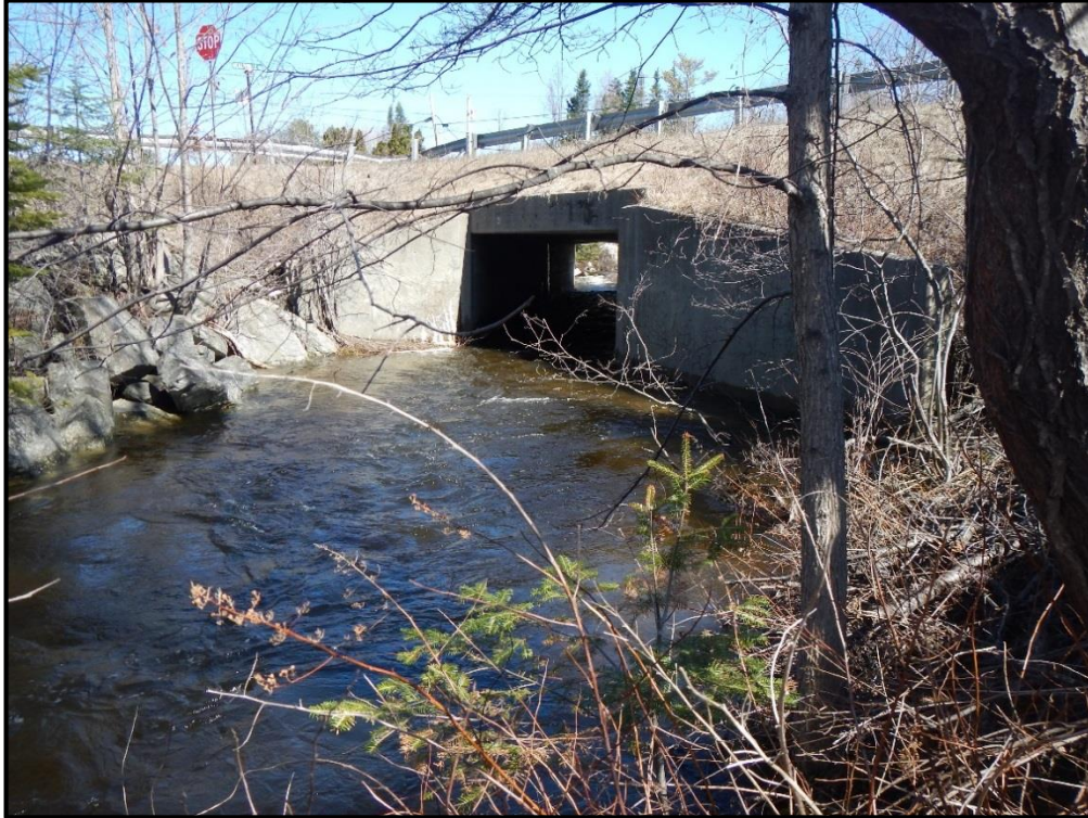
T-MH-S-14 Culvert Outlet
