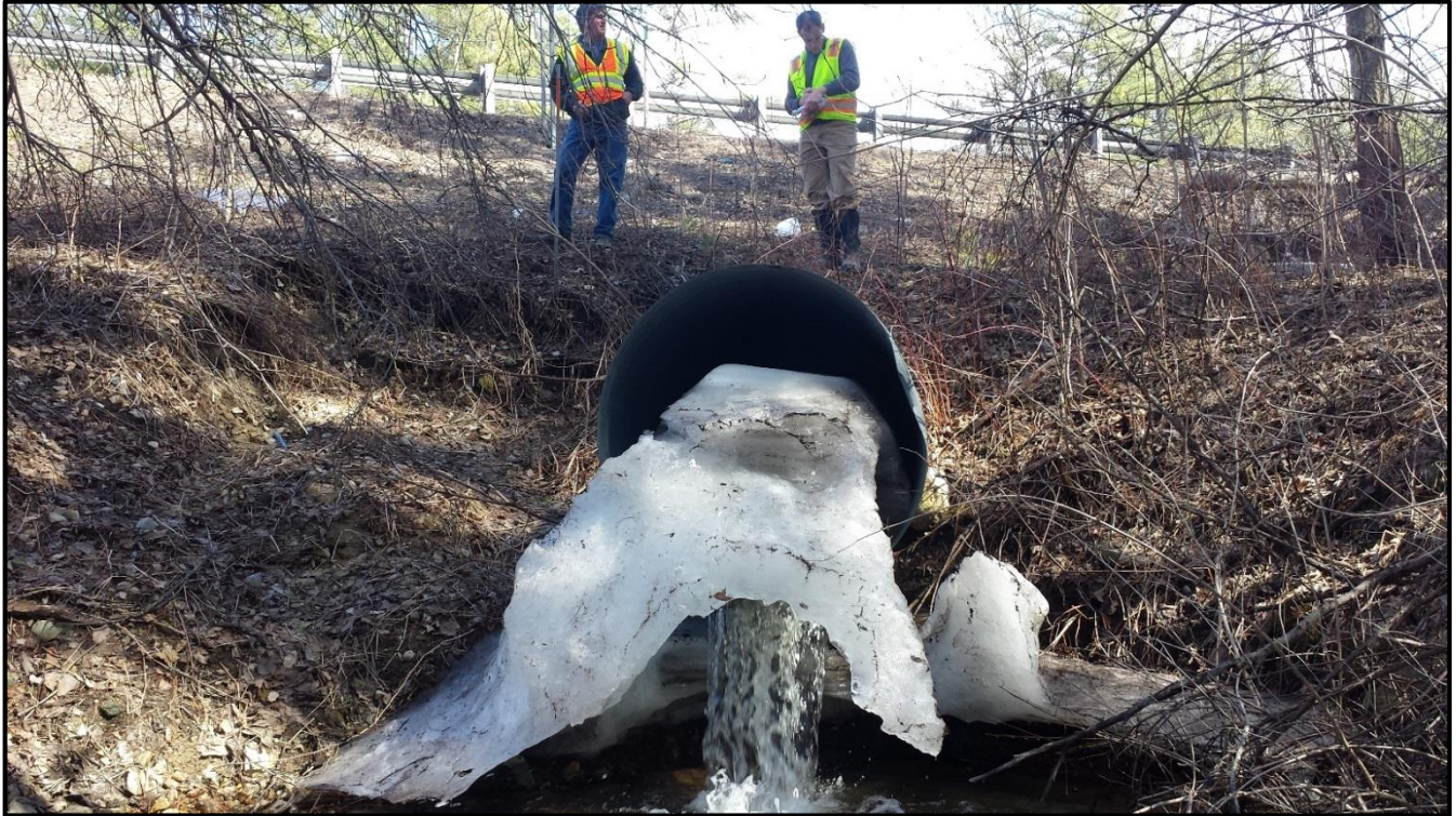
T-CL-S4 Culvert Outlet / Downstream Channel
