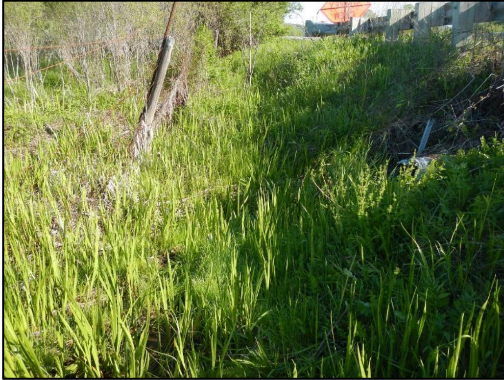
V-BE-S-100 Culvert Inlet / Upstream Wetland V-BE-AW-100
