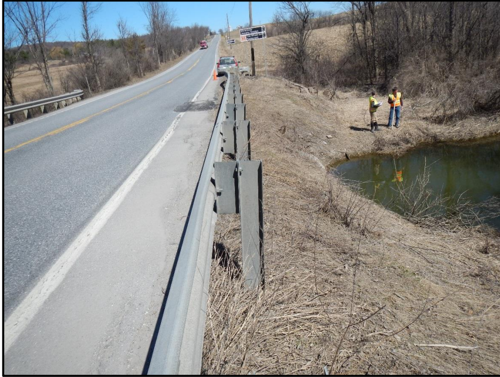
V-BE-S-102 Down Station Roadway along Route 22A (North)
