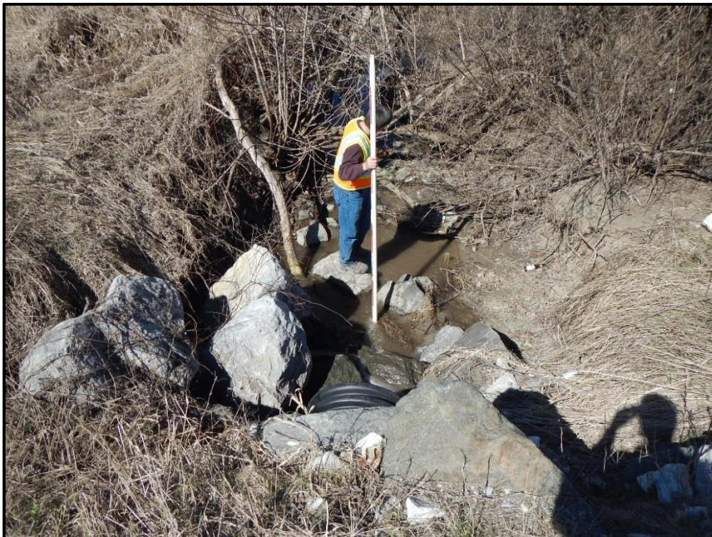
V-BE-S-109 Downstream Channel
