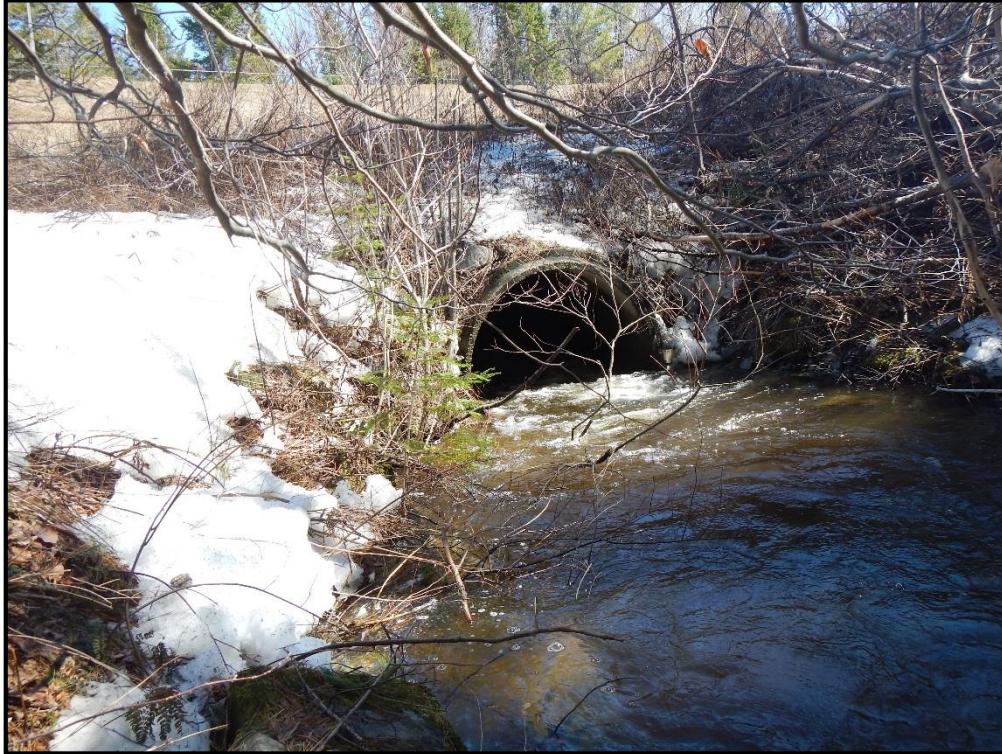
T-MH-AS-20 Culvert Outlet
