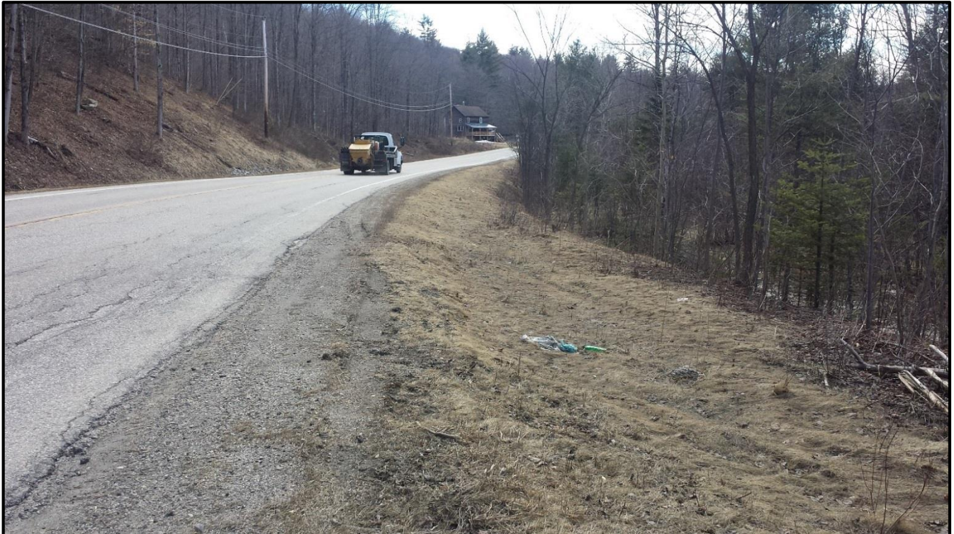
V-WA-S106 Up Station Roadway
