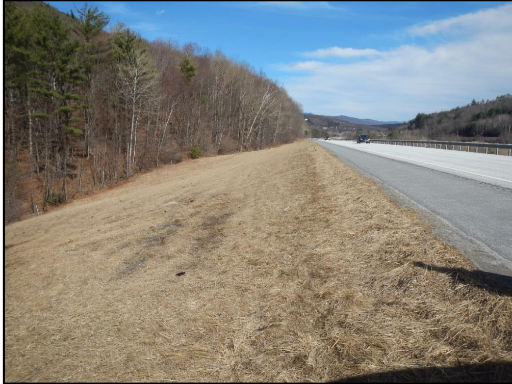
T-WR-S34 Down Station Roadway
