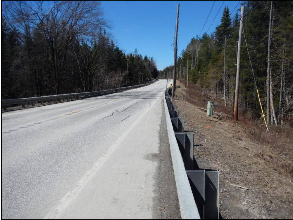
T-MH-S28 Down Station Roadway
