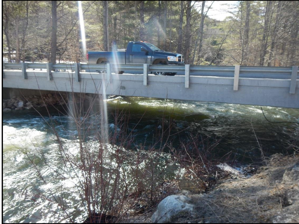
T-LU-S1 Upstream Face of Bridge
