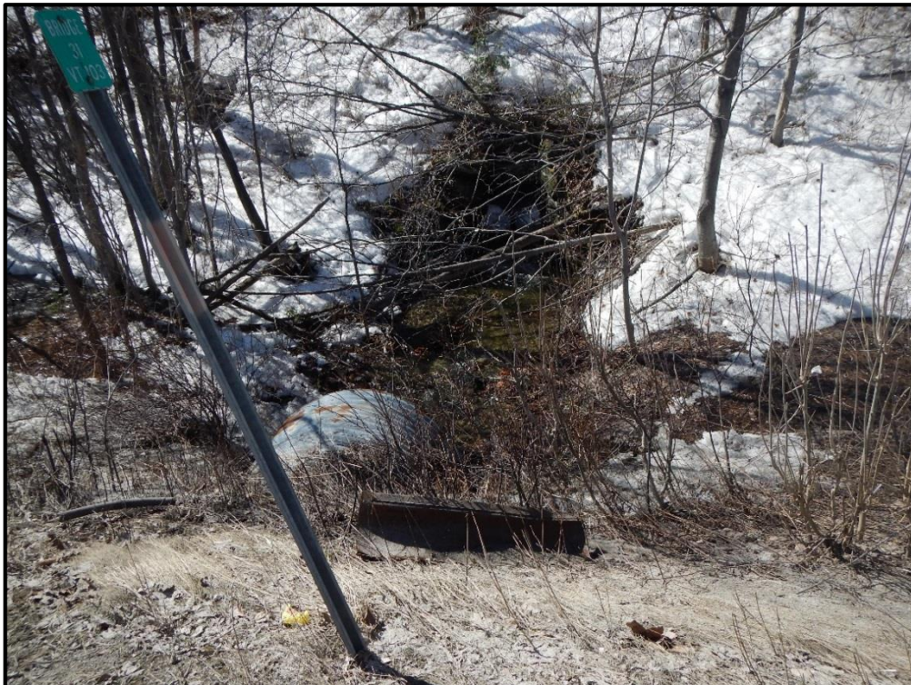
T-MH-S1 Upstream Channel
