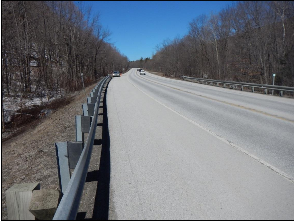
T-MH-S1 Down Station Roadway
