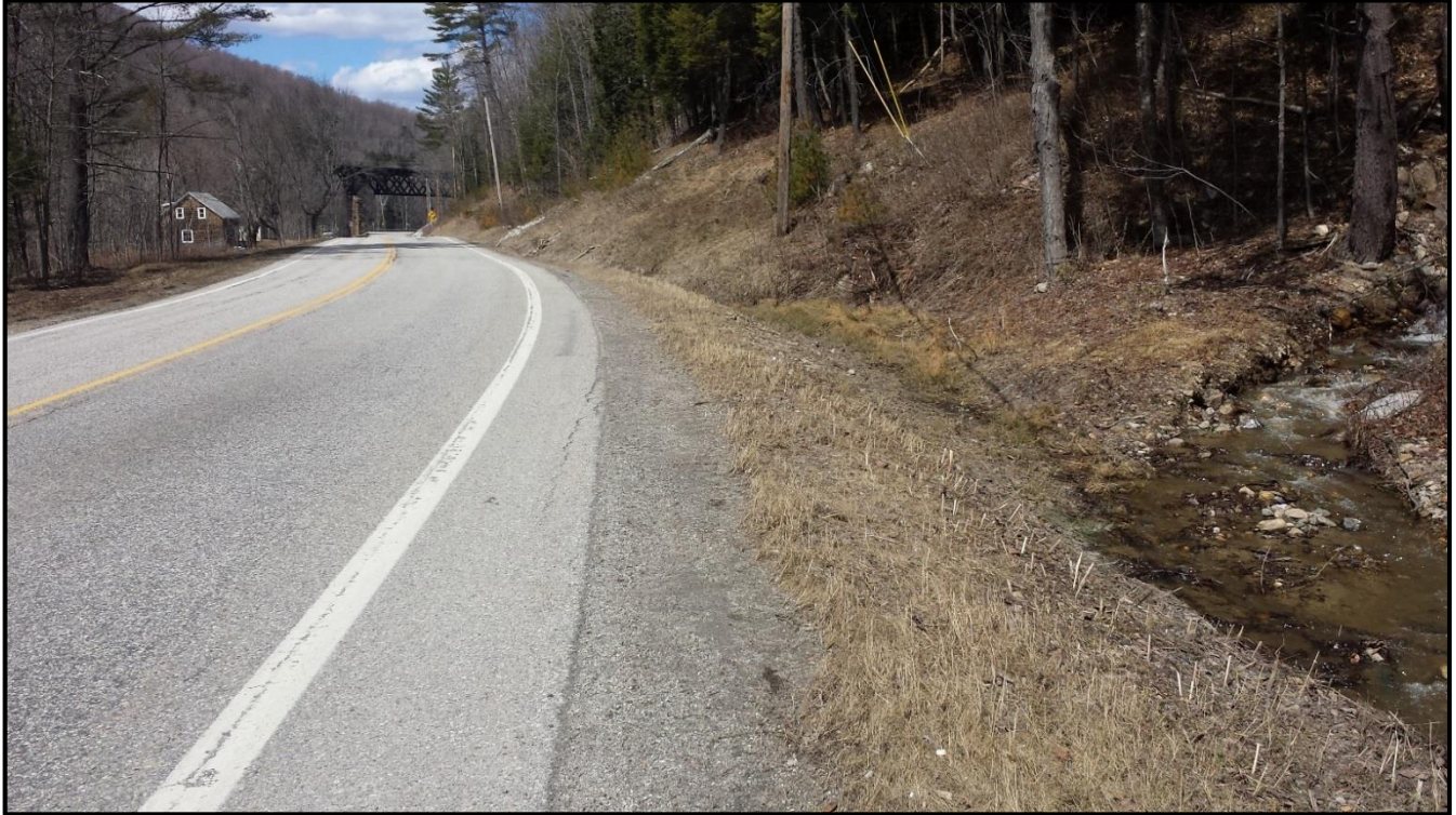
V-WA-S106 Down Station Roadway
