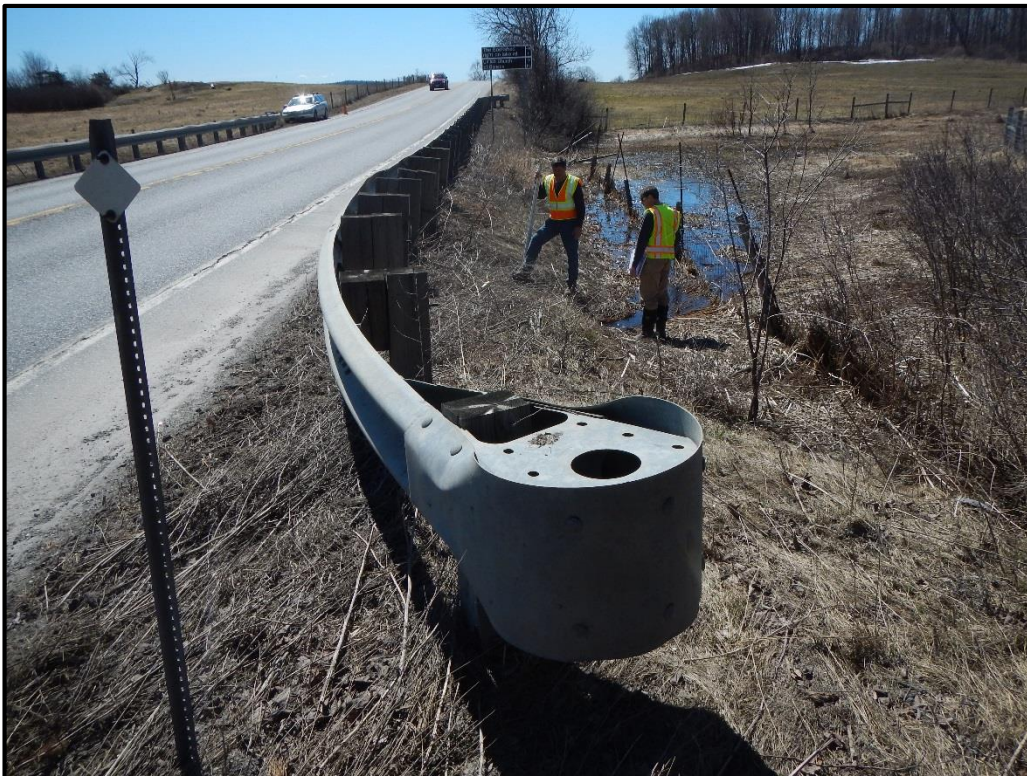
V-BE-S-100 Inlet Upstream View
