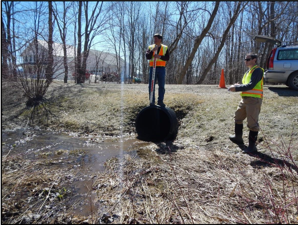
V-BE-AS-10 Culvert Inlet / Upstream Wetland (V-BE-AW-17)
