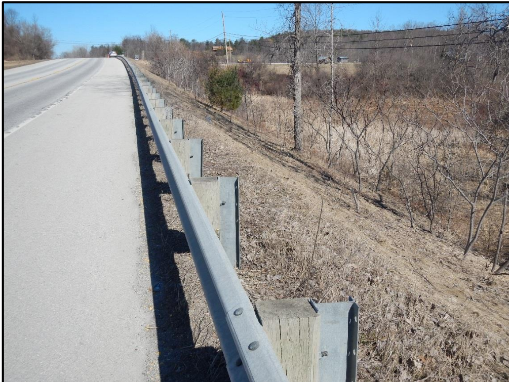
V-FH-S-17 Down Station Roadway
