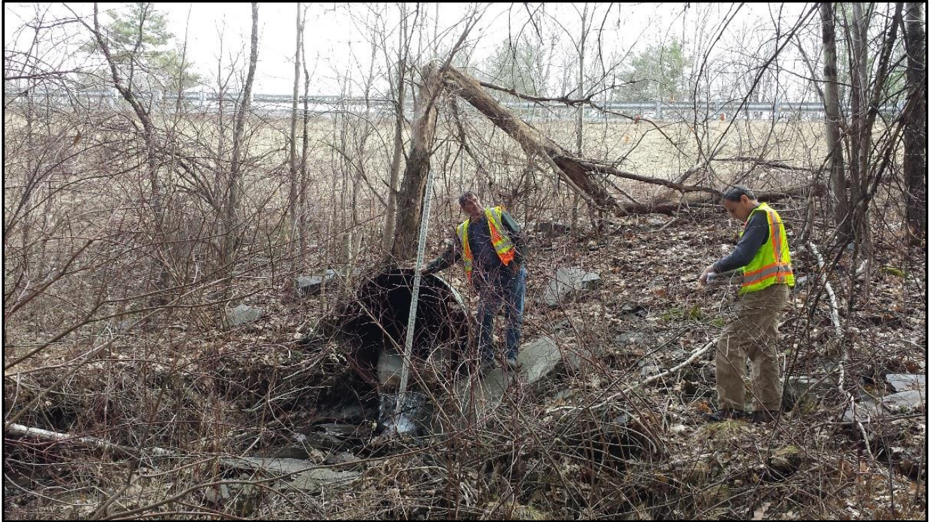
V-FH-S-5 Culvert Outlet
