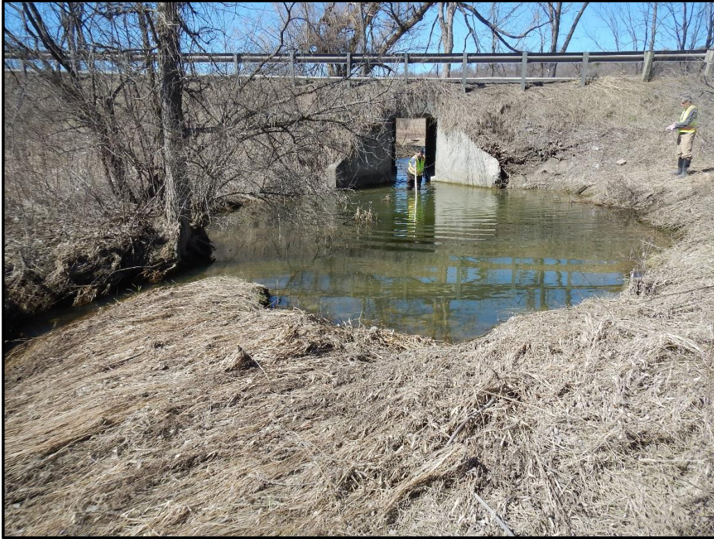
V-BE-S-102 Culvert Outlet
