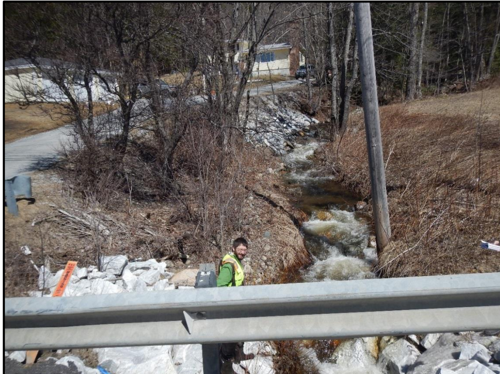
T-MH-S37 Upstream Channel
